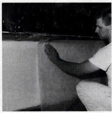
Specification Chemicals' Nu-Wal system is used to restore cracked plaster walls.
