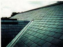
The Top Slate system of ridges, hips and vents from Castle Metal Products is designed to strengthen the weakest areas of slate roofs.
