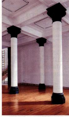
The old-growth heart pine flooring was remilled by Goodwin Heart Pine and installed in the oldest building in Key West, FL, to match the existing flooring.
