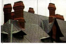
Kronenberger & Sons' restoration of the exterior of the Mark Twain House in Hartford, CT, included masonry raking and repointing, as well as replacing the chimneys following a corbelling design found in historical photos.
