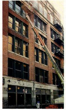
Armakleen used ARMEX®, a baking-soda based medium, to clean the Boydel Building in Detroit, MI.
