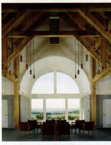
The Vermont Veterans Memorial Chapel in Randolph, VT, was built by Vermont Timber Works using natural and glue-laminated timbers and traditional mortise-andtenon joinery.
