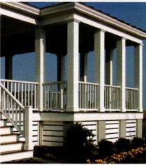
HB&G's PermaWrap columns in cellular PVC and other porch parts offer durability and weather resistance.
