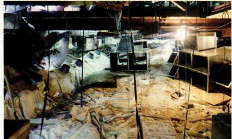
Above: In the summer of 1996, holes were cut in the roof over the auditorium of the academy so steel trusses could be introduced to take the load off the original wood trusses, some of which had begun to check dangerously. To provide workers with enough room to assemble the steel trusses, temporary platforms were suspended between each pair of timber trusses in the cramped attic space, shown here.
