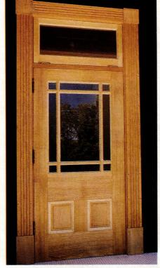
To build this raised-panel door and entryway, Weston Millwork used 2-in.-thick, solid-edge grain sugar pine.
