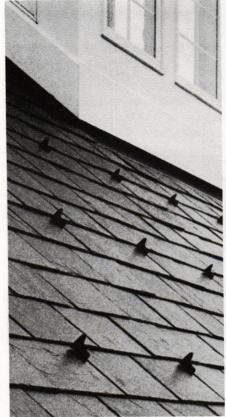
Cast bronze snow guards in a variety of patterns for slate, tile, and shingle roofs are the specialty of MULLANE SNOW GUARDS. Write in No. 56
