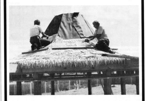
At last, the demand has been met for a thatch that is virtually indestructible. Tropic Top™, a lightweight metal shingle, colorfast, 100% fireproof, installs as easily as ordinary roof shingles, and has the appearance of natural thatch without any of the disadvantages.
