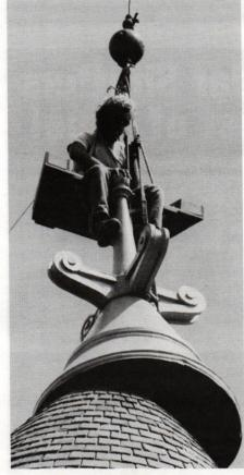
MIDLAND ENGINEERING CO. refurbished and reinstalled 4 turret caps at the University of Nortre Dame's 1889 Sorin Hall. The sheetmetal caps, historic ornamentation that had never been properly maintained, suffered serious deterioration due to rust, bird excrement, and lightning. Write in No. 742
