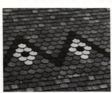
CERTAINTEED produces premiumgrade, extra-thick asphalt shingles in colors and shapes that can create the look of traditional slate, shingle, and tile roofs. Write in No. 754
