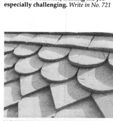
The batten-seam copper roof on the 28-ft.-dia. Bergen County, N.J., courthouse was fabricated and installed by VULCAN SUPPLY. The 22 curved battens tapered both in width and thickness, making the job
