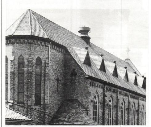
Concrete roof tiles, manufactured to closely resemble the colors and textures of natural slate, were used to re-roof this historic church. The Early American Slate tiles were produced by VANDE HEY RALEIGH. Write in. No. 284
