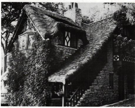
C&H ROOFING first won national attention for its steam-bent cedar shingle roofs that resemble thatch. The firm now works internationally and installs virtually any traditional roof — from natural thatch to standing-seam copper. Write in No. 743
