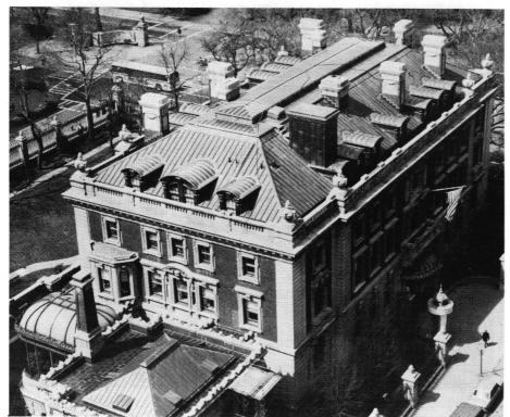
NIKO CONTRACTING CO. replicated the original copper roof — and associated architectural copper work — on the Cooper-Hewitt Museum in New York City. The firm also had to replace all the wood decking and repair concrete decking, some structural steel, drain lines, and some interior plaster. Write in No. 830
