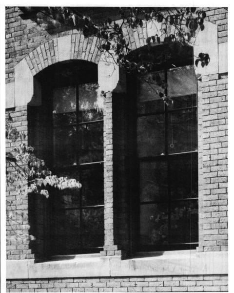
Architectural Components, Inc., fabricated this replacement window in Eastern white pine and mahogany sash, insulated glass, and 1-in. muntin bars for Weld Hall, Harvard University.
