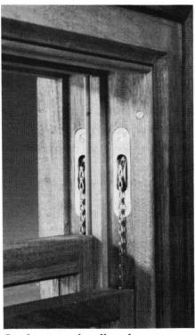
Cast bronze sash pulleys, bronze weatherstripping, copper-dipped sash chain, and stop moldings held with brass screws seated in brass grommets for stop adjustments are typical details in a custom window from WOOD WINDOW WORKSHOP. Write in No. 964
