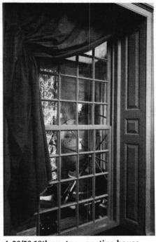
A 20/20 18th-century meeting house window with Restoration Glass built by ARCHITECTURAL COMPONENTS, INC., along with interior storm with insulated glass. ACI also built the raised-panel wainscotting, window seat, and associated millwork.
