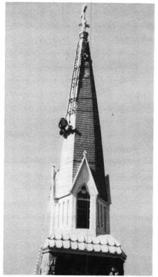
A steeplejack with The JACK HASSLER COMPANY replaces missing slate on the steeple of St. Dominic Catholic Church in Philadelphia.
