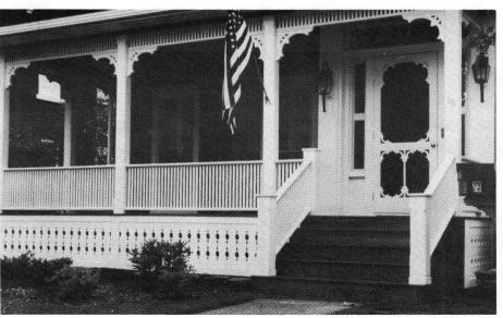
Complete porch parts were done by J.A. DAWLEY FINE WOODWORKING: Brackets and porch skirt were custom made; posts were splined, then chamfered; and the railing system was designed to direct water away from seams. Write in
