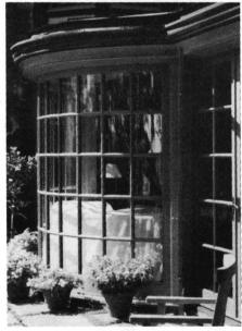
The manufacturing flexibility of ZELUCK DOORS & WINDOWS that enables it to engineer almost any shape window is demonstrated on this custom bow-front true-divided-lite residential window. Write in No. 692
