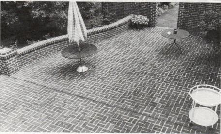
DOMINION RESTORATION specializes in mild masonry cleaners that avoid the use of mineral acids. In the top photo, "Bio-Cleanse" is used to remove dirt, mold, and mildew from brick pavers (the reaction with organic matter turns the material white.) After a 20-minute soak, a water wash leaves the brick completely clean. Write in No. 231
