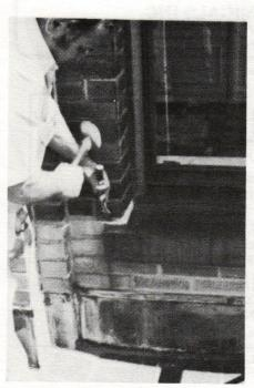
A craftsman from GENERAL RESTORATION CO. removes existing deteriorated sealant from construction joints, prior to recaulking with a longlife acrylic terpolymer sealant. Write in No. 238
