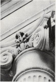
After installation of NIXALITE, a stainless steel needle strip, prime perching spots like the tops of capitals and architraves no longer attract pesky birds. Write in No. 37
