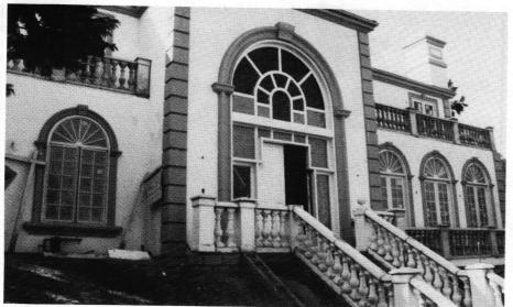
Balustrade and exterior ornament cast in Forton MG (polymer-modified gypsum); supplied, along with technical support, by BALL CONSULTING  $Write\ in\ No.\ 726$
