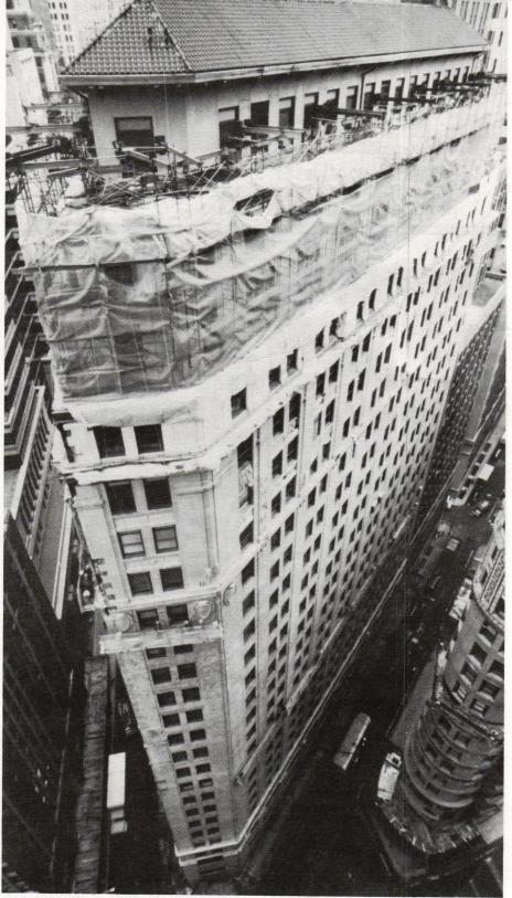
On this major commercial building, AOI WATERPROOFING is replacing approximately 2,000 terra cotta units with pre-cast concrete and GFRC on two cornice bands. Write in No.~45
