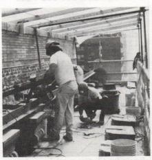
On this university building, craftsmen from RESTORATION CONCEPTS are engaged in a cornice restoration/ rebuilding project: Steel armatures cleaned and repaired, new steel shelf angle put in place, and new cast concrete elements and salvaged terra cotta masonry installed. Write in No. 319
