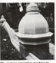
The contour generating machine in the mill of BRIAR HILL STONE CO. permits economical cutting of custom jobs. Shown above is the upper replacement cornice, bonnet, and lower cornice in cut sandstone, fabricated for the restoration of Meadowport Arch, Prospect Park, Brooklyn, N.Y. Write in No. 89
