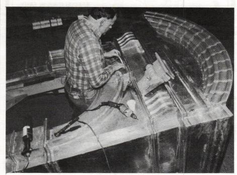
Bill Steinmetz Jr. of MIDLAND ENGINEERING is fabricating new dormers from Wolmanized plywood and lead-coated copper for the Hamilton County Courthouse in Noblesville, Ind. Write in No. 742
