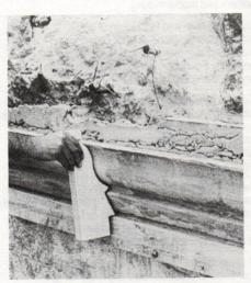
Exterior molding is repaired with Conpro-set — a polymer-modified all-purpose patching cement that can be shaved to final form. CONPROCO makes a wide range of masonry repair and restoration products. Write in No. 481
