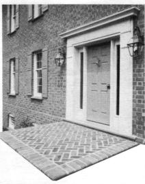
This front stoop is made of standard size "Old Williamsburg" in a herringbone pattern with half round bullnose step stread and 8X8 in. corners. OLD VIRGINIA BRICK Write in No. 90
