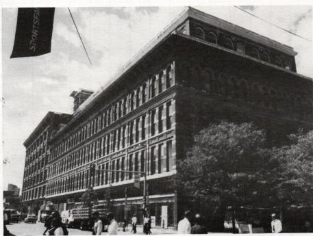
The historic brickwork and limestone trim of the Denver Dry Goods building, in downtown Denver, CO, had disappeared under a dozen layers of hazardous lead-based white paint averaging 1/8" thick. After extensive testing, it was found that the PEEL AWAY 1 system from DUMOND CHEMICALS would remove all the layers of paint in one application, while safely keeping all the lead-paint safely contained on the peel-off cloth. Write in No. 590
