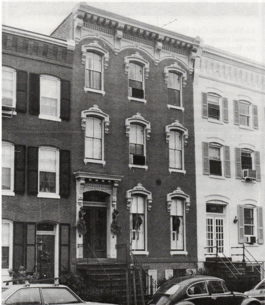
Facade of Brown's 1870 townhouse in Washington's Capitol Hill historic district. The stoop contains the area's only surviving brownstone steps; the facade had been less well treated, and Brown had to replace missing window-hood brackets, cresting, and balconies and to hand-scrape white paint off the facade.
