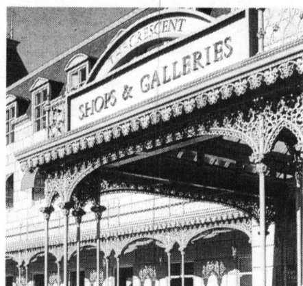
HISTORICAL ARTS & CASTING , a high-end, custom cast-metal foundry fabricated this spectacular aluminum canopy (finished with a fluoropolymer coating) installed in a Dallas commercial property. Write in No. 121
