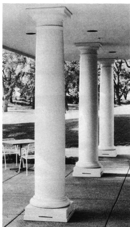
Massive wood columns in the Tuscan order were fabricated for this covered patio by PAGLIACCO TURNING & MILLING. Write in No. 707
