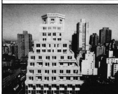
This architect chose FRP cornice over cast stone on the East 87th Street Apartments in New York City.
