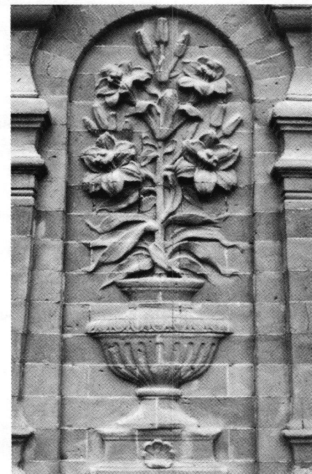
A late Victorian building embellishment in carved and rubbed brick on the exterior of a London town house.
