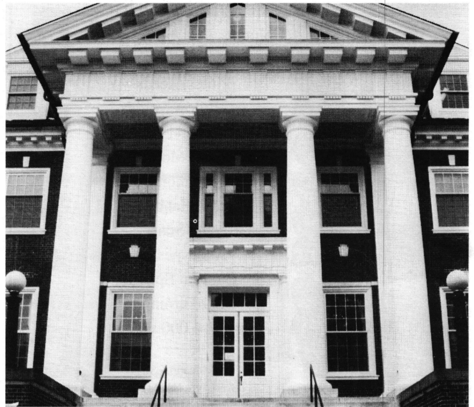
Columns for this impressive Doric entry were engineered and fabricated in FRP by EDON CORP. Write in No. 189
