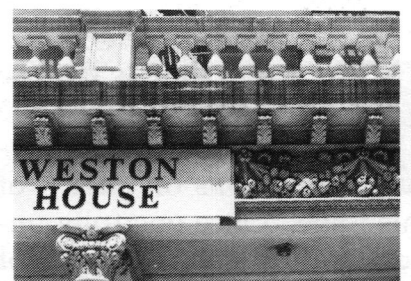
FRP used at exterior of Weston House, N.Y.C.
