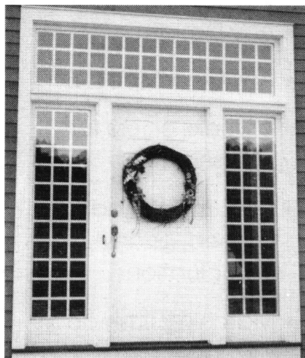
New entry for Colonial-style house was designed by WOODSTONE COMPANY, using their computer modeling system to scale up dimensions from the historic original without altering the proportions.
