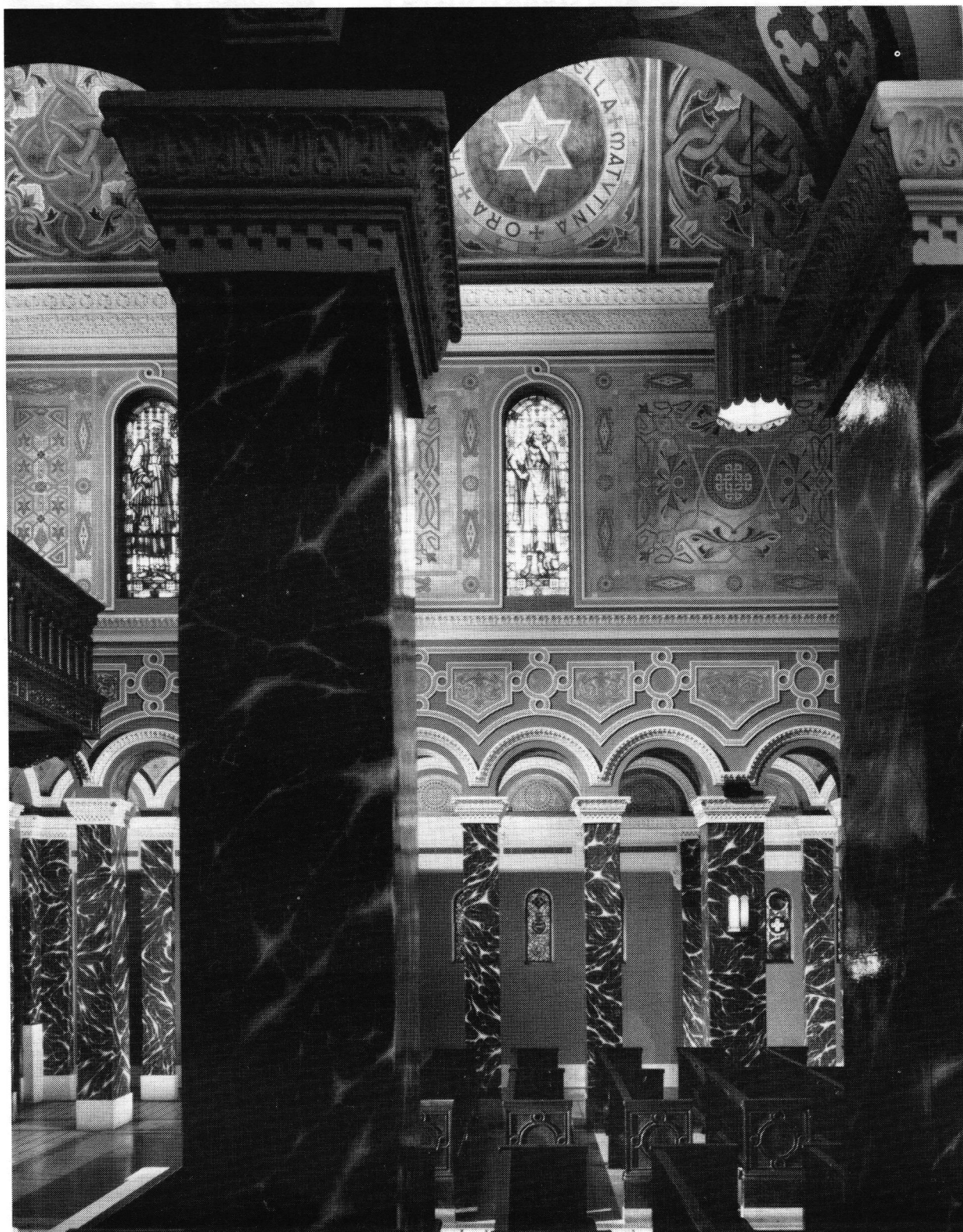
Johnson's new lighting emphasizes St. Clements' lavish restored stencilwork, from the ceiling to the arch soffits. Octagonal overhead fixtures designed by Johnson direct metal halide light upward and incandescent downward.
