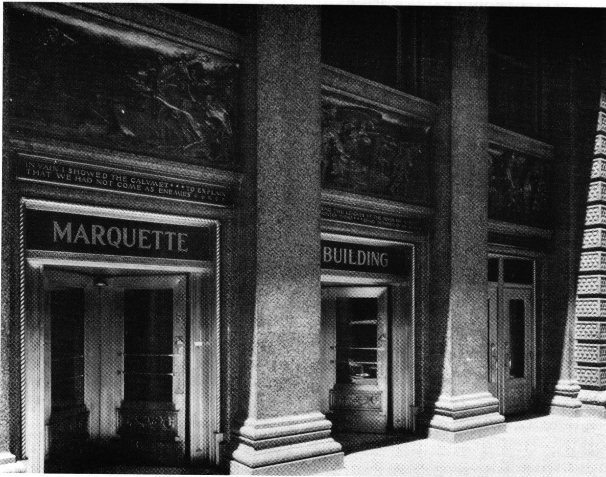
The Marquette Building was designed by Holabird and Roche, the predecessor firm to Holabird & Root, Walker Johnson's employer throughout his career. He oversaw the restoration of bronze bas reliefs and revolving doors at the entrance as well as the terra-cotta and cast-aluminum trim on the storefronts.
