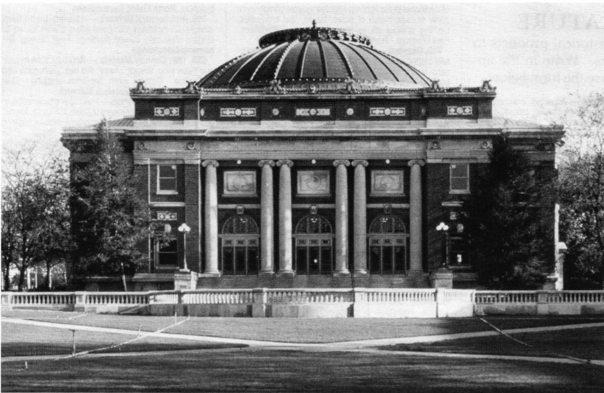
Improving a faded structure's image with new illumination is a Johnson specialty. At the University of Illinois' Foellinger Auditorium, acoustics were bad but, the structure beloved. Johnson reworked the interior for better sound, shored up an unsound roof by adding a backstage wing, and strung lights along the dome's ribs.
