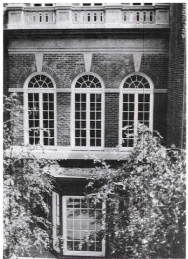
The rear elevation, which overlooks the back garden, uses carved limestone elements to punctuate the red brick. A copper-sheathed bay window provides additional space and light for the ground floor
