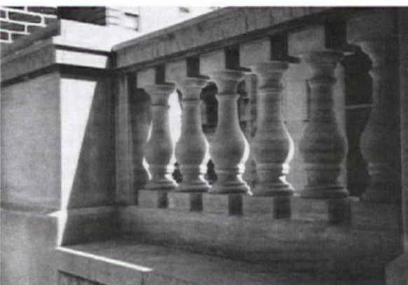
Detail of the new carved limestone balustrade that crowns the facade in front of the set-back which starts at the fourth-story level
