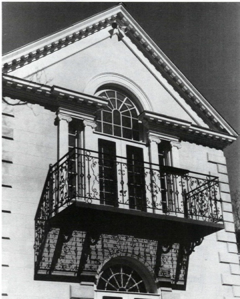
A Palladian window and ornate iron balcony grace the facade of the house
