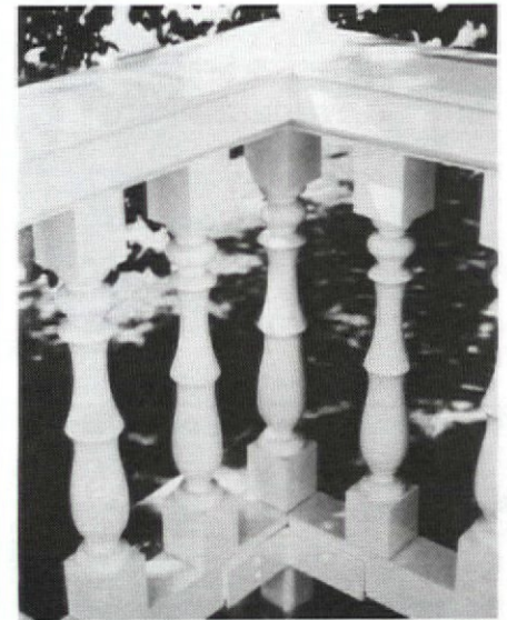
Close-up of balusters recreated as part of the reconstruction of the Hamilton County Bandstand in Aurora, Nebraska. SACO MANUFACTURING & WOODWORKING
