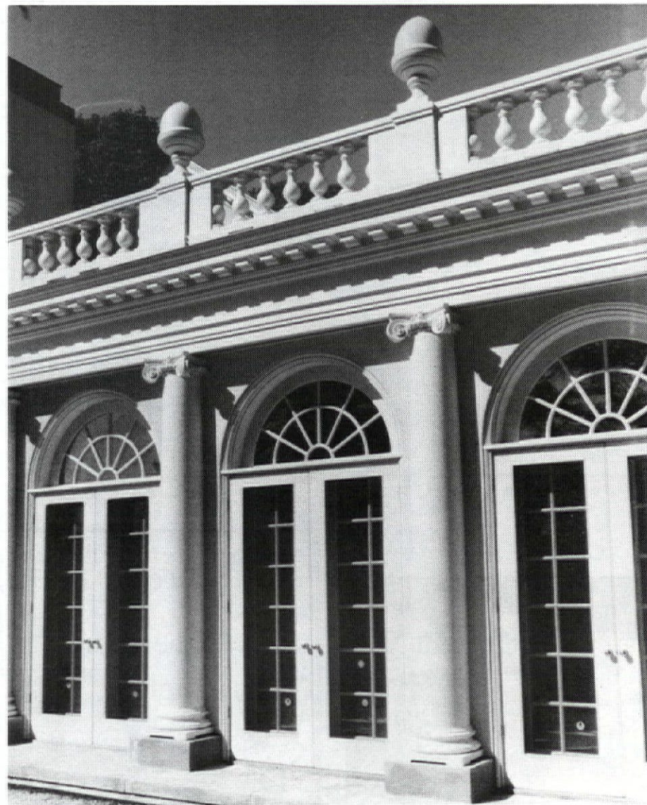
Stone acorns cap the roof balustrade
