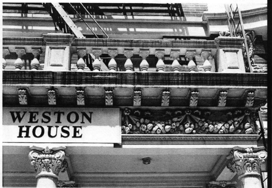
FGRP used at exterior of Weston House, N.Y.C.
