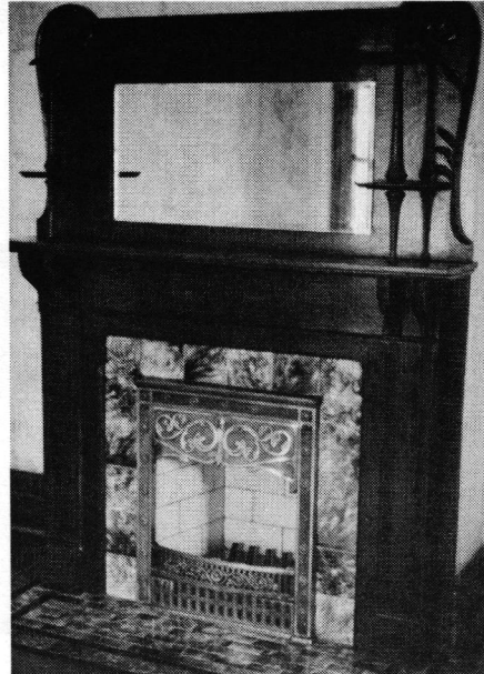
■ 1895 coal fireplace converted to Rumford fireplace, for added radiant efficiency. "Rumfordizing" involves rebuilding firebox and flue, and is well suited to retrofitting tall Victorian fireplaces. Buckley Rumford Fireplace Co. , Box 21131, Dept. TB, Columbus, OH 43221 (614) 221-6131. Write in No. 553
