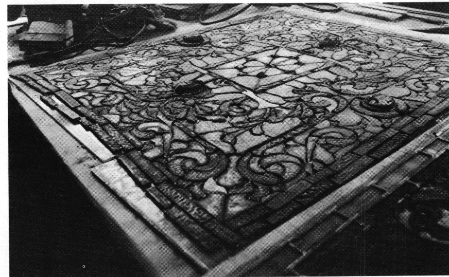
■ One of 12 Victorian 30-by-40-in. stained-glass windows the company has restored. Third-generation studio's typical commissions include ecclesiastical, commercial, and residential buildings. Pike Stained Glass Studios , 180 St. Paul St., Dept. TB, Rochester, NY 14604 (716) 546-7570. Write in No. 791
