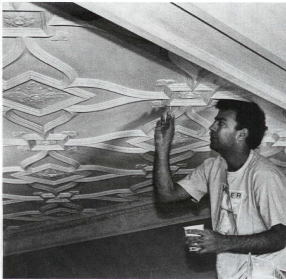
Plaster restoration in Connecticut residence. Art Home
