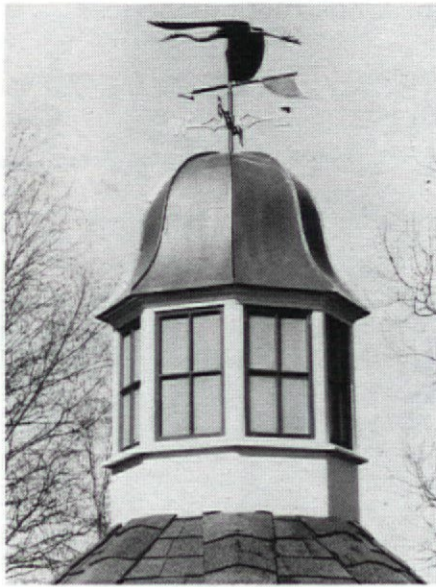
Frosted-glass windows and standing-seam copper roof grace a wood cupola by Denninger Cupolas & Weather Vanes
