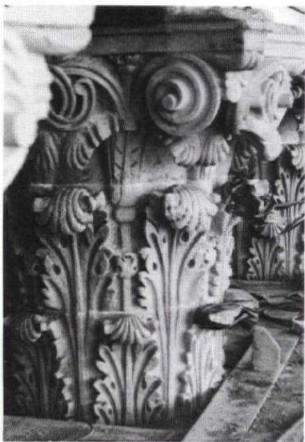
Carved limestone Corinthian capital restored for the State Capitol in Topeka, Kansas by Smither Studios
