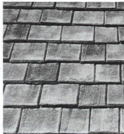
Handmade Hendrick concrete tile from Richmond Precast Concrete Products have been used at Colonial Williamsburg to simulate wood shingles while adhering to fire codes
