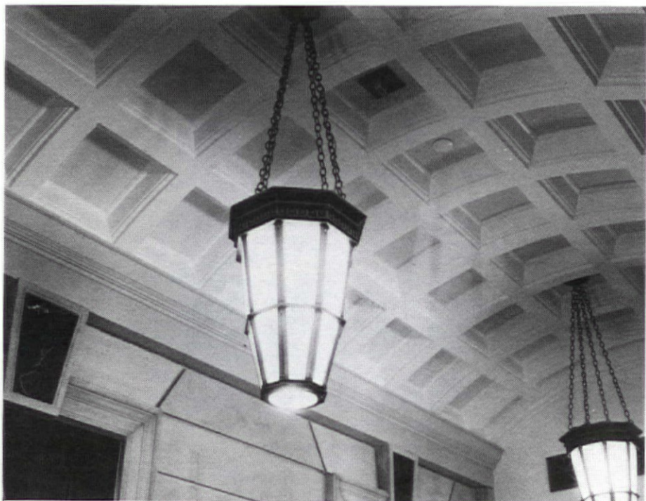
Vaulted Ceiling, Sweeney Building, Brooklyn, NY
