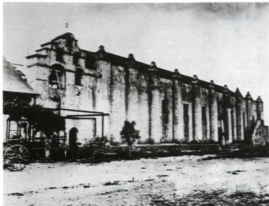
Green is designing invisible seismic bracing for the San Gabriel Mission, one of California's oldest buildings
