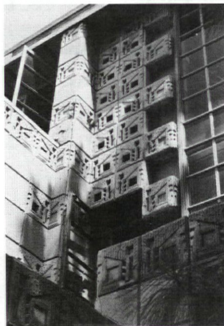
Frank Lloyd Wright pioneered cast-stone "textile blocks" on the Freeman House in L.A.; Green is reinforcing the building without spoiling its character
