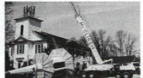
Landmark Rigging at work on the Norfield Congregational Church
