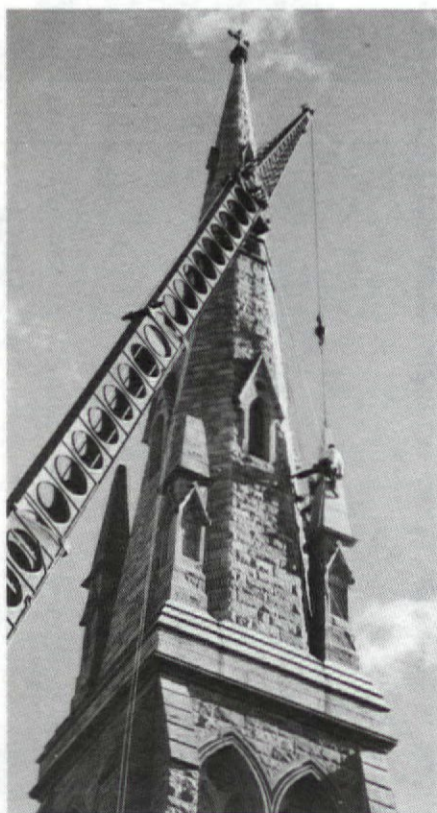
Architectural Timber & Millwork at work on a masonry steeple
