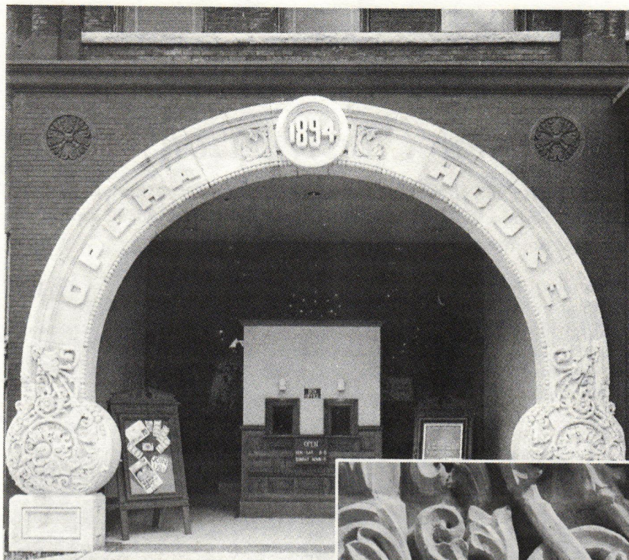
A carved limestone entry arch announces the date of construction of the Grand Opera House in Galveston. (Photo: Van Edwards)
