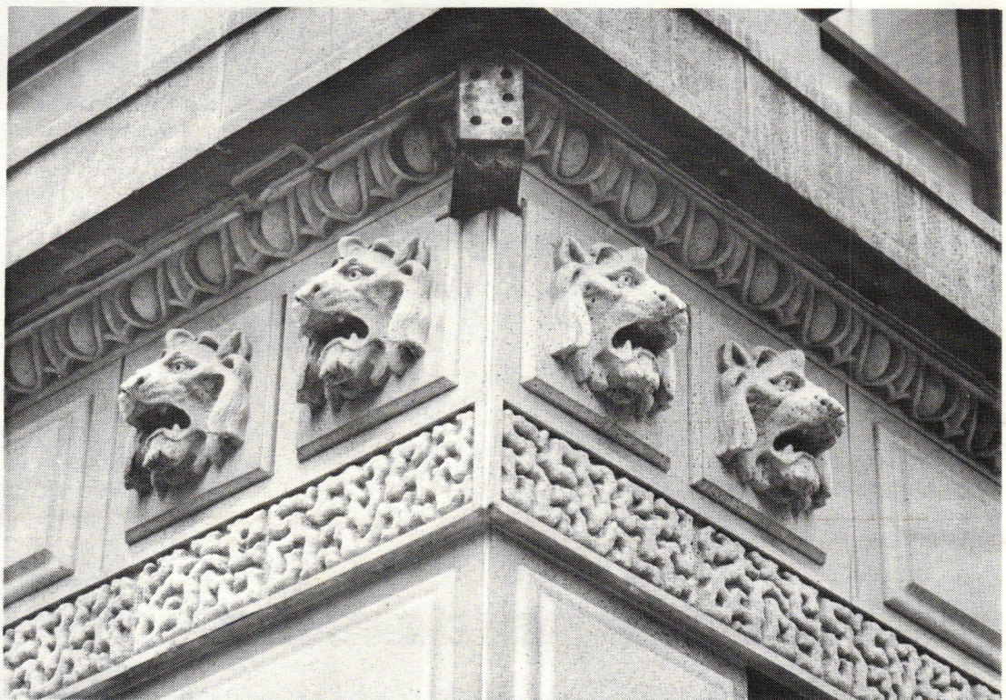
▲ Above: GFRC, INC., created these GFRC panels that replicate an original terra cotta frieze. ▼ Below: This cast-aluminum acroterion, over 10 ft. high, was produced by HISTORICAL ARTS & CASTING for the Field Museum in Chicago.
