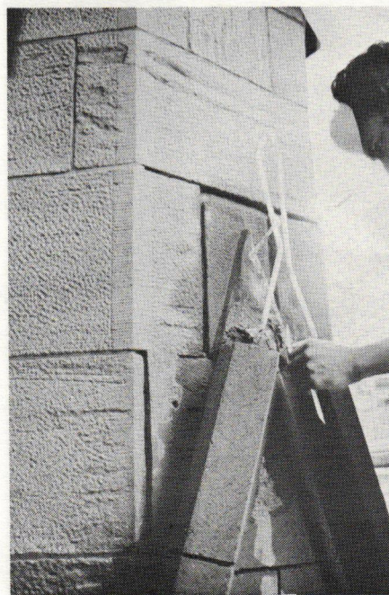
For large protruding patches, armatures are used to reinforce the Jahn patching material. Threaded nylon rods are inserted into 1/4-in. dia. holes drilled 3/4-in. deep on 4-in. spacings. Rods are glued into the holes with a polyester adhesive. Nylon armatures are kept at least 3/4 in. below the finished surface of the patch.
