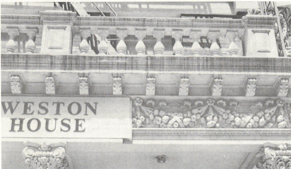
▲ Above: The entablature and parapet of this building was replaced using cast stone custom-fabricated by MJM STUDIOS. ▼ Below: FRP moldings from ART HOME STUDIO were used to restore this hotel portico.
