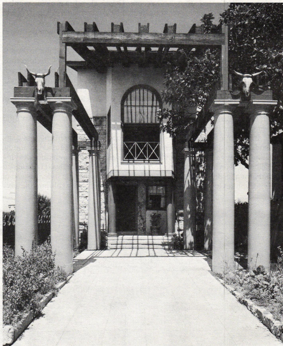
Three-dimensional bucrania hang above the Doric columns on this Richmond, Calif., residence by Thomas Gordon Smith, dean of the architecture school at the University of Notre Dame. The rough-hewn entablature and timber beams reflect native California architecture. Limestone sheaths the house; marble pilasters flank the door; and the plants are descendants of those cultivated in ancient Roman gardens.
