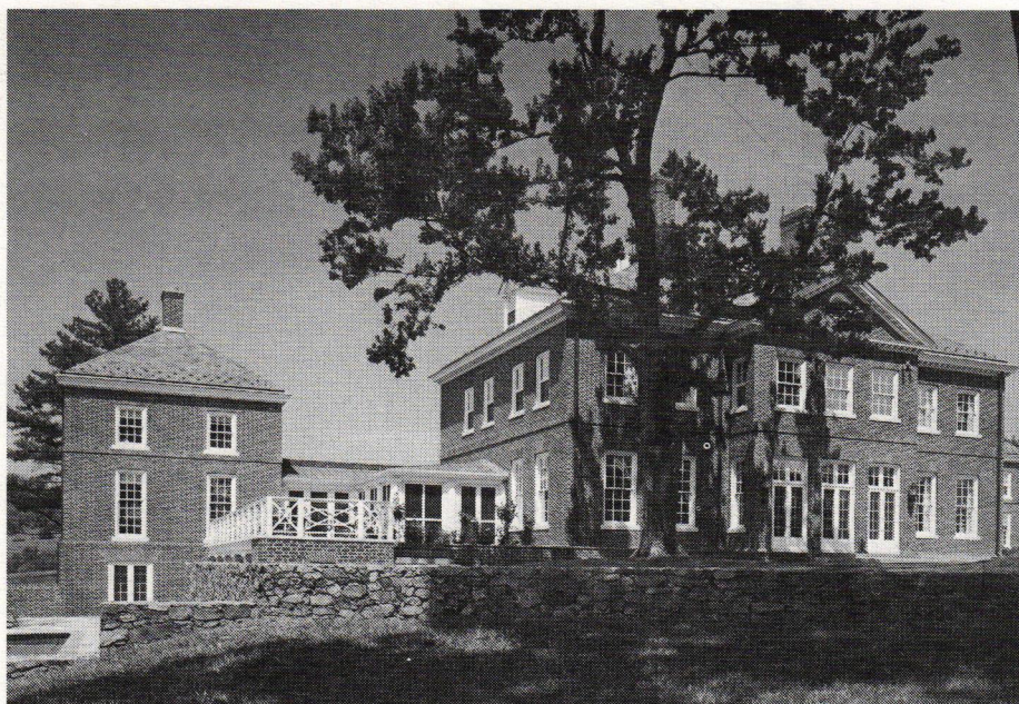
Tony Atkin & Associates of Philadelphia produced the Georgian country house in Virginia (shown), which has two symmetrical hip-roof wings. Just visible at right is the garage wing and at left is a sitting room and office wing. The French doors illuminate a library. The bricks are handmade; slate covers the roof. (Tony Atkin, principal in charge of design; Cameron Mactavish, project architect; Daniella Holt Voith, Bill DuPont, David Genthur, and Ruth Rowe, staff. Tony Atkin & Associates is the successor firm to Tony Atkin, Architect, and Atkin, Voith.)
