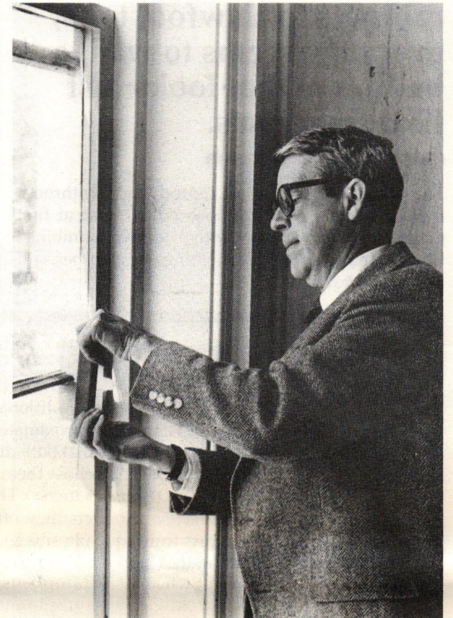
Harvie Jones records a muntin profile in the 1848 McDowell house in Huntsville to add to his personal archive of documented historic buildings.
