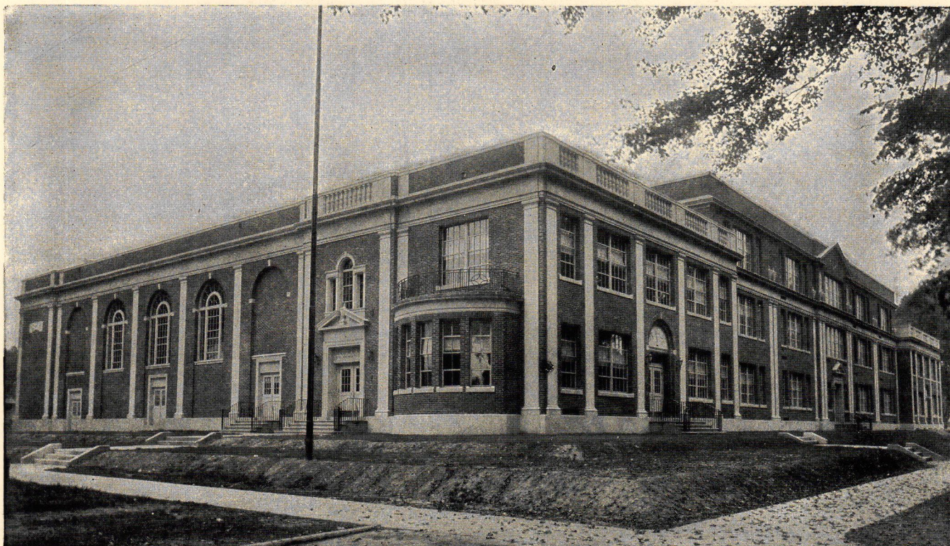
Architect: Carl C. Ade, Rochester, N. Y. WATERLOO HIGH SCHOOL Htg. Contractor: Warnock & Zahndt, Rochester, N. Y.
