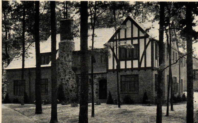
In the home of Mr. Joseph H. Skaggs of Atlanta, Georgia, provision for complete telephone convenience is made by nine telephone outlets, including one in the servants' quarters over the garage. FRAZIER & BODIN, Architects, Atlanta, Georgia.
