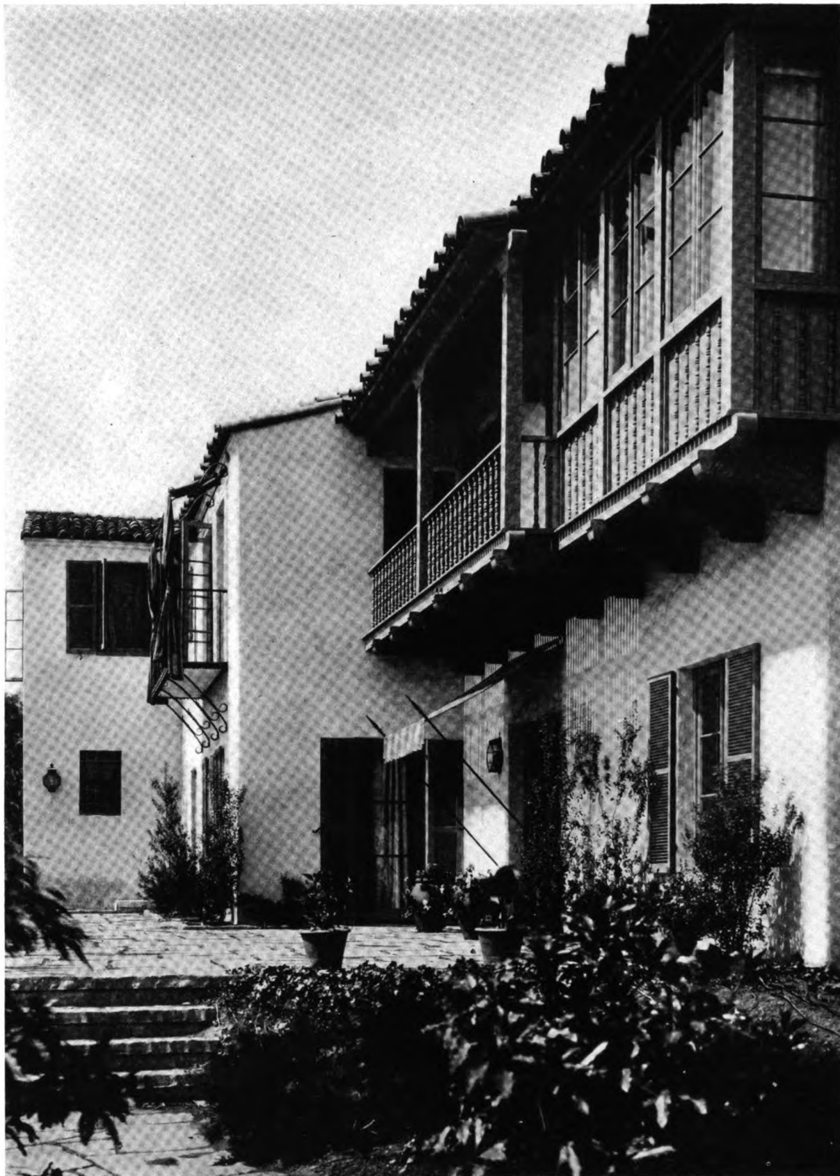
Gordon B. Kaufmann, Los Angeles, Architect Terrace Front, House, Dr. Edwin Janss, Los Angeles, Calif. Photograph taken especially for The Architect—never before published
