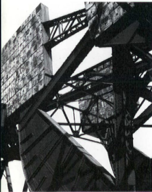
Old Colony Bridge, Boston. Built by Schertzer Rolling Lift Co., 1898. While the imperative of the bridge was to ameliorate the conflicting patterns of rail and water traffic by use of a pivoting mechanism, the bridge designers created some of the most elegant formal, visual relationships to be found anywhere in Boston's built environment. Photo © Peter Vandewarker.
