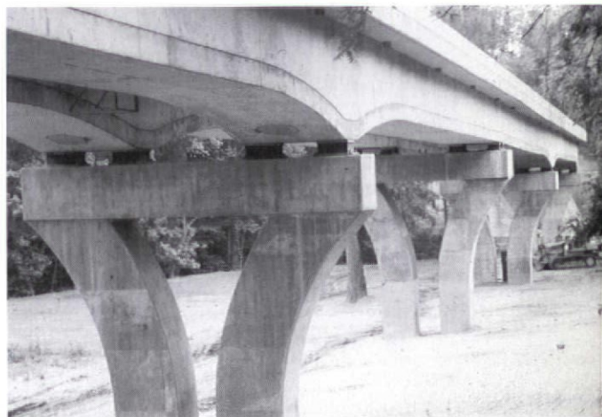
MetroLink bridge piers and superstructure. Courtesy Bi-State Development Agency.
