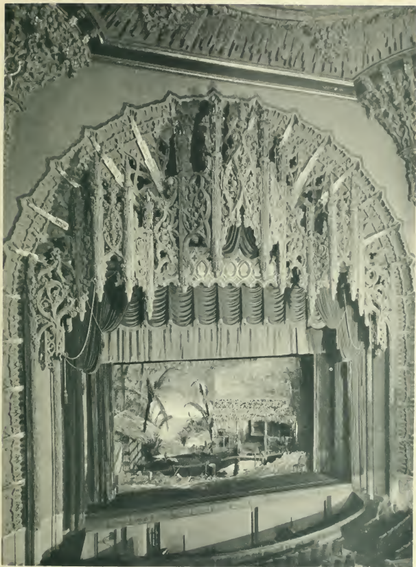
PROSCENIUM ARCH, UNITED ARTISTS THEATER, LOS ANGELES, CALIFORNIA. WALKER AND EISEN AND C. HOWARD CRANL, ARCHITECTS.
