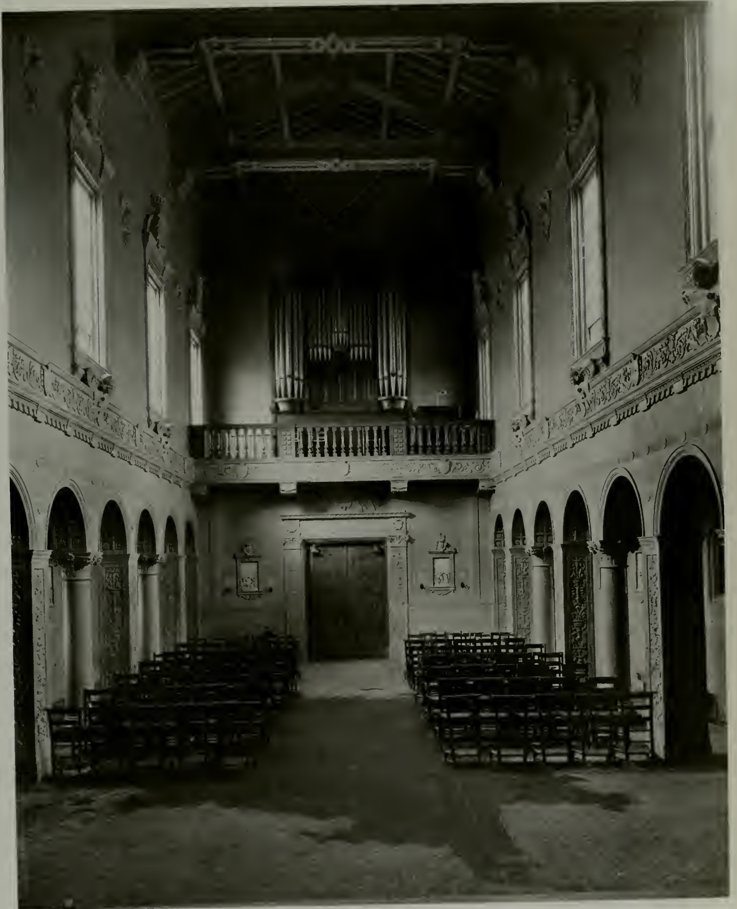
INTERIOR OF CHAPEL, LOOKING TOWARD ENTRANCE CARMELITE MONASTERY, SANTA CLARA, CAL. MAGINNIS & WALSH Architects
