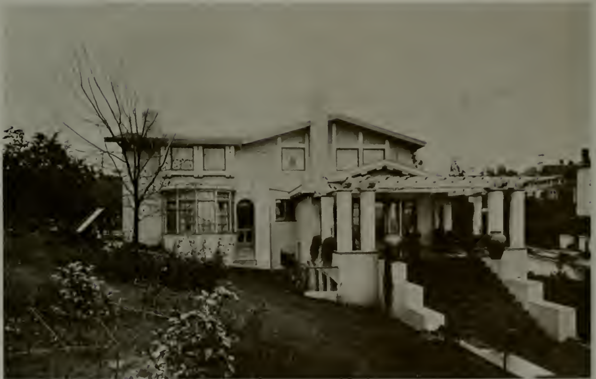
WEST (GARDEN) VIEW RESIDENCE OF STANLEY DOLLAR, OAKLAND, CALIFORNIA CHAS. W. McCALL, Jr., Architect
