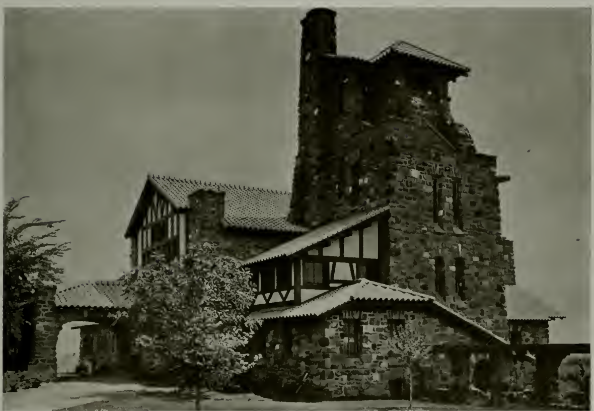
TOWER END FROM UPPER LEVEL RANCH HOUSE, YAKIMA, WASHINGTON WILLIAM M. KENYON, MAURICE F. MAIZE, Architects
