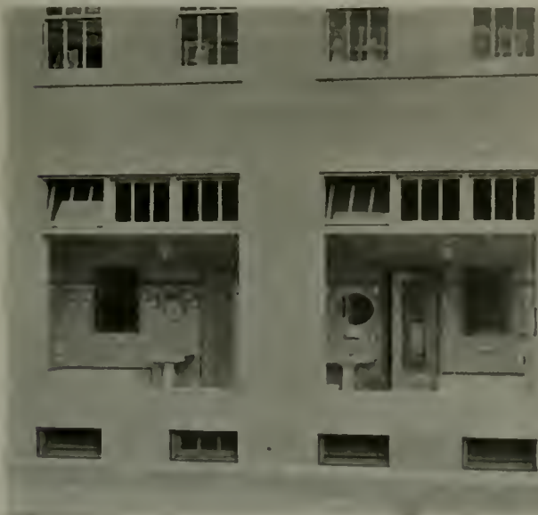
EXTERIOR DETAIL, OAKLAND BRANCH
