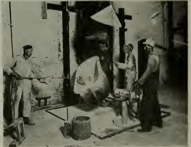
SIFTING ENAMEL ON A RED-HOT BATH TUB
