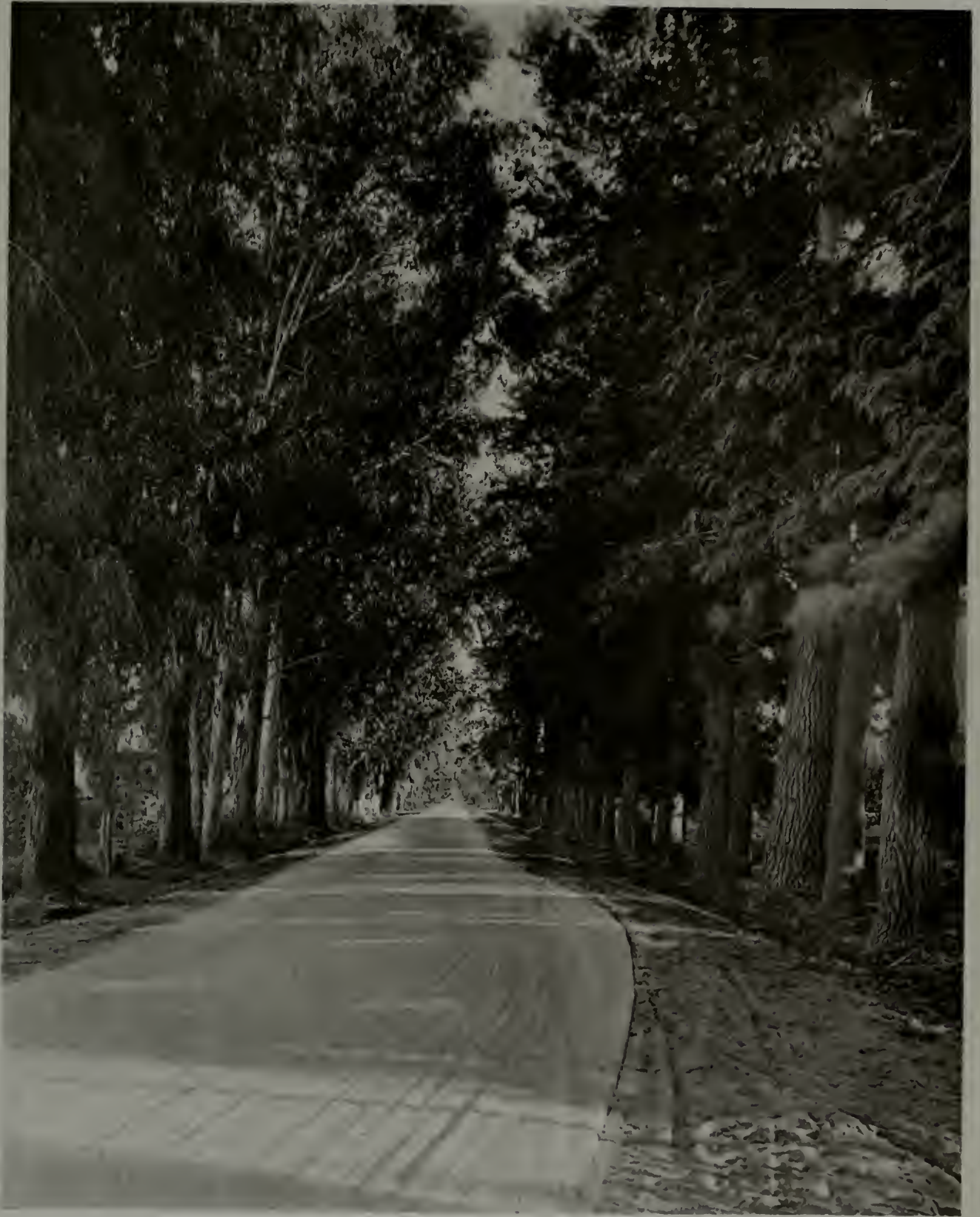
BOULEVARD—SANTA ANA ROAD SAN DIEGO STATE HIGHWAY
