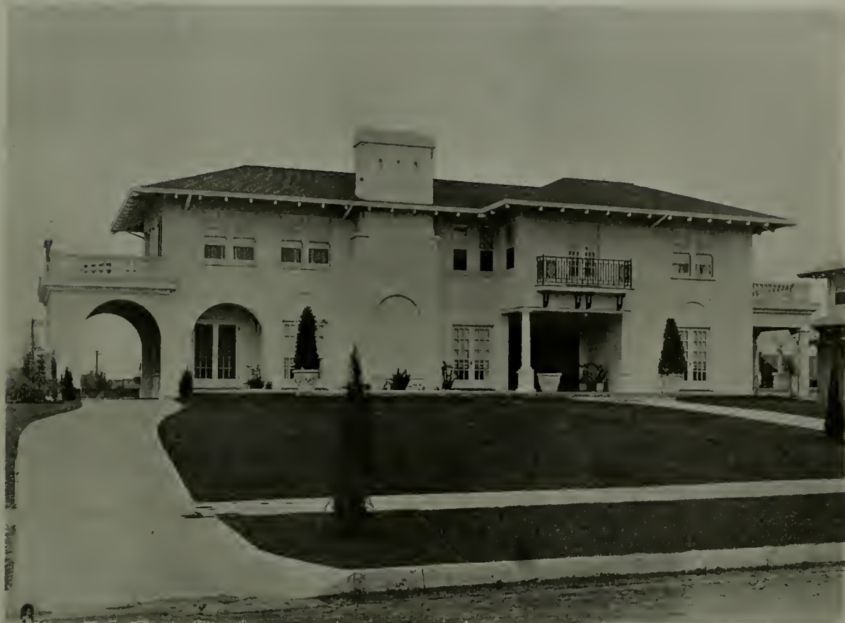
A.—THE CONSISTENCY OF THIS VIGOROUS COMPOSITION IS INJURED BY THE TREATMENT OF MAIN ENTRANCE PORCH
