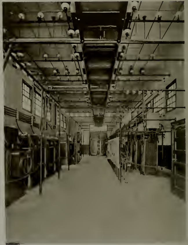
LOS ANGELES No. 1 SUB-STATION
