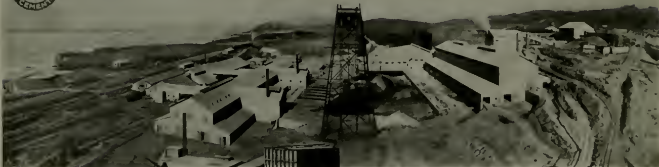
GENERAL VIEW OF PLANT
