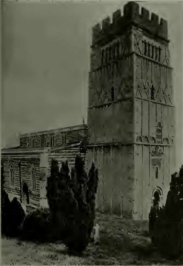
TOWER, EARL'S BARTON CHURCH
