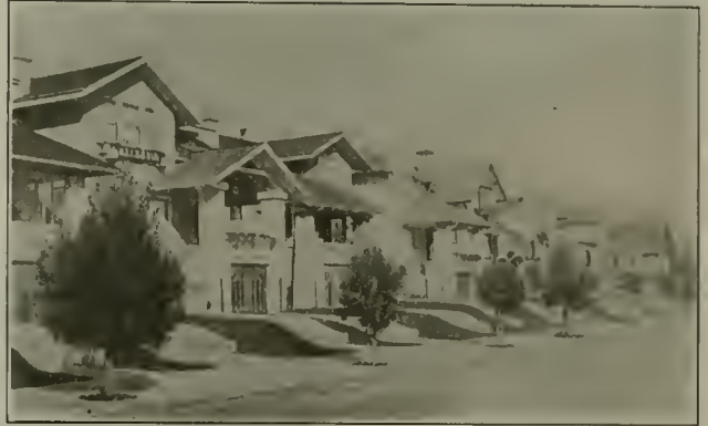
NEW CONSTRUCTION IN WEST PORTAL PARK
