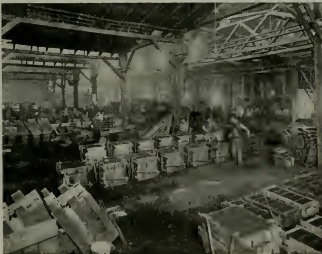
MAKING CASTINGS FOR ENAMELED IRON WARE
