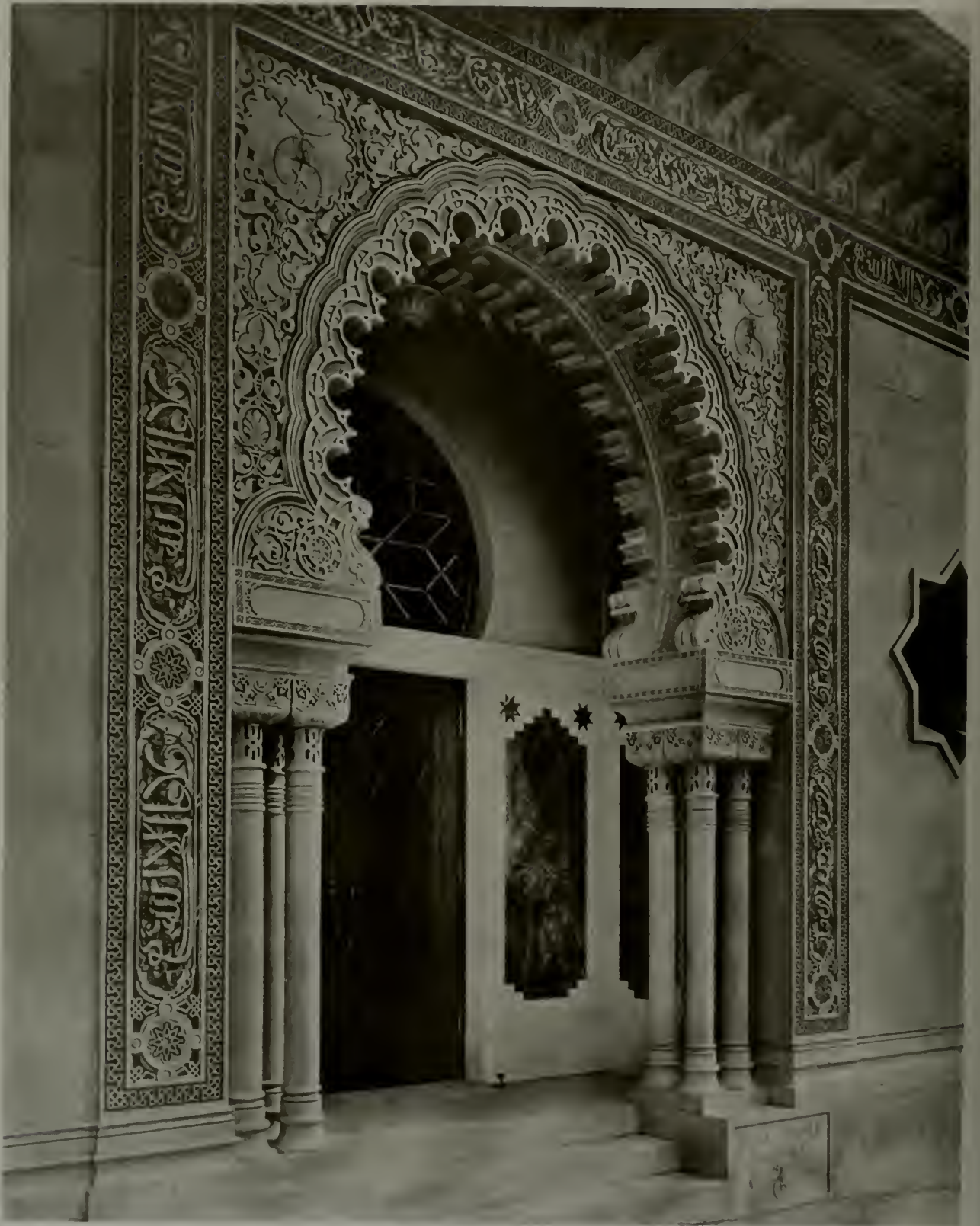
ENTRANCE ISLAM TEMPLE, SAN FRANCISCO T. PATERSON ROSS, Architect
