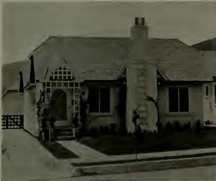
D.—THIS STURDY LITTLE HOUSE IS WEAKENED BY THE SMALL SCALE OF ITS CORNER TRELLIS
