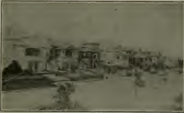
NEW CONSTRUCTION IN WEST PORTAL PARK
