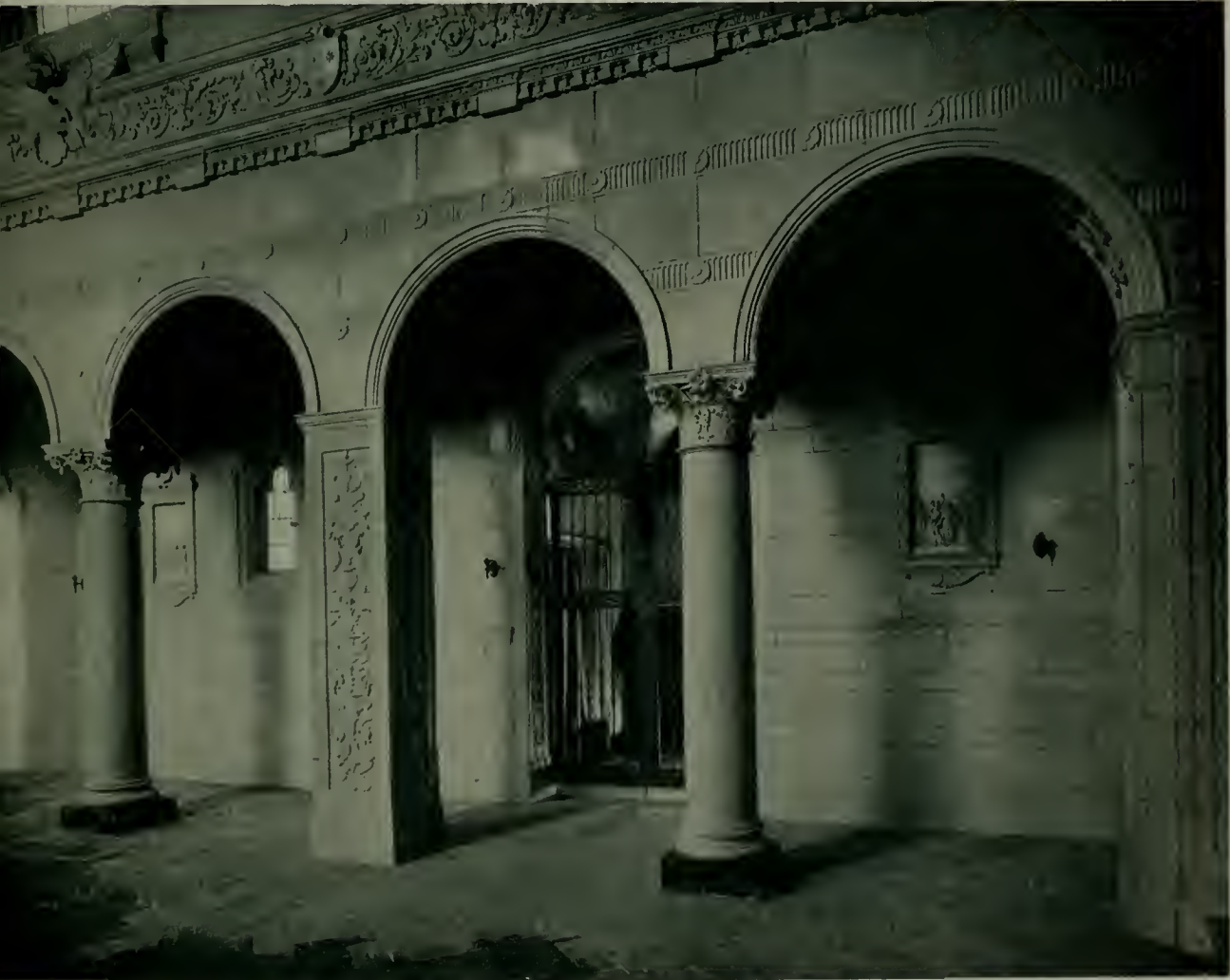
CHAPEL DETAIL AND ENTRANCE TO LADY CHAPEL CARMELITE MONASTERY, SANTA CLARA, CAL. MAGINNIS & WALSH, Architects
