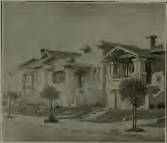
NEW CONSTRUCTION IN WEST PORTAL PARK
