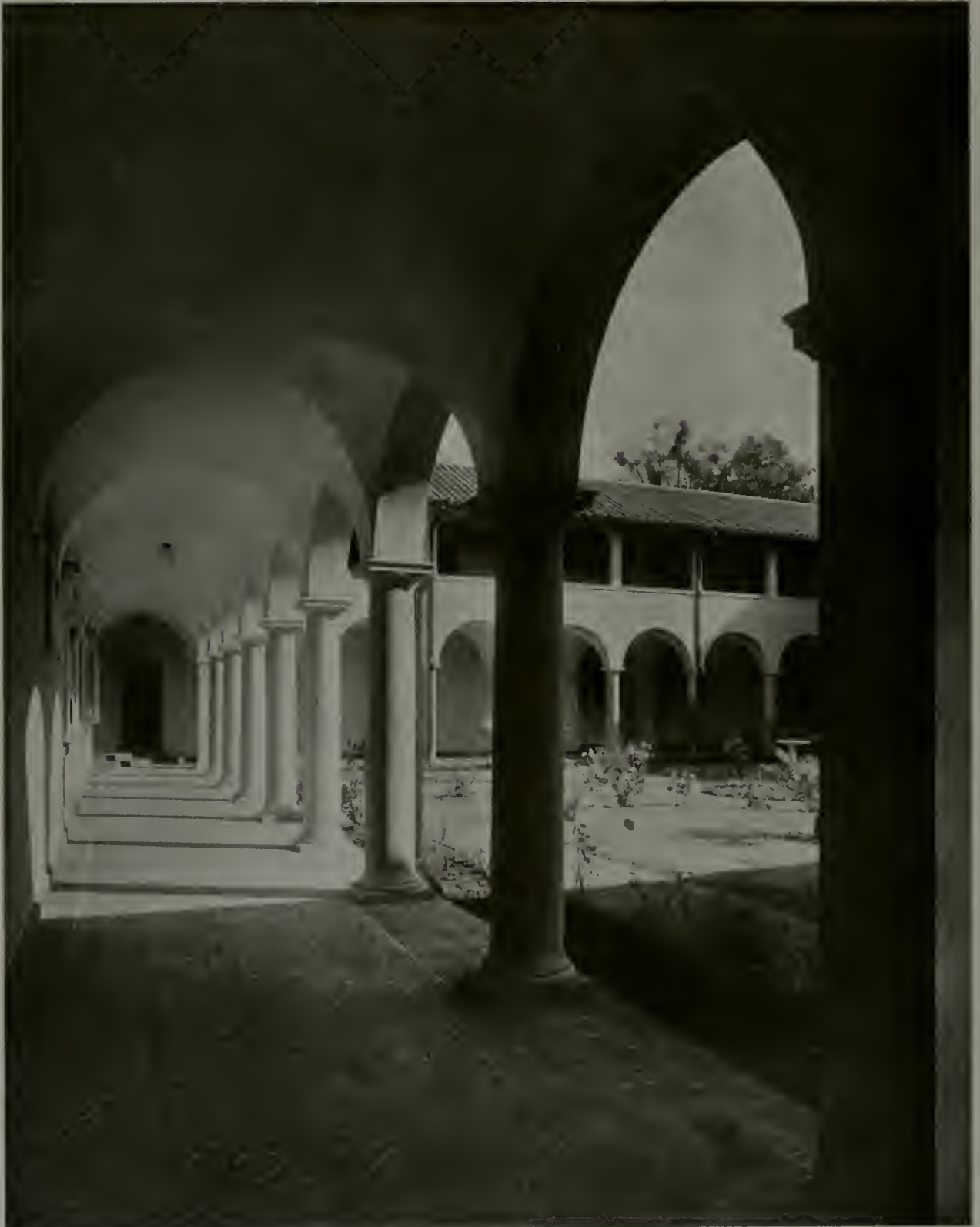
LOGGIA IN CLOISTER CARMELITE MONASTERY, SANTA CLARA, CALIF MAGINNIS & WALSH, Architects
