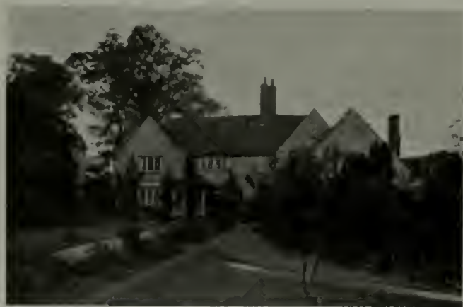
C.—THE DOMESTIC QUALITY OF THIS HOME IS EMPHASIZED BY THE IRREGULAR GABLES AND GROUPS OF SMALL-PANED SASH.
