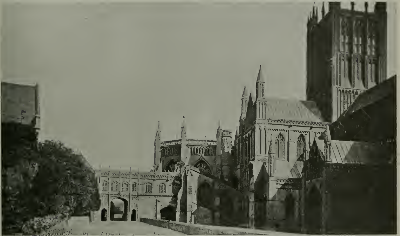
NORTH VIEW, SHOWING CHAPTER HOUSE AND CHAIN GATE
