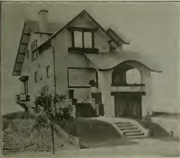
NEW CONSTRUCTION IN WEST PORTAL PARK
