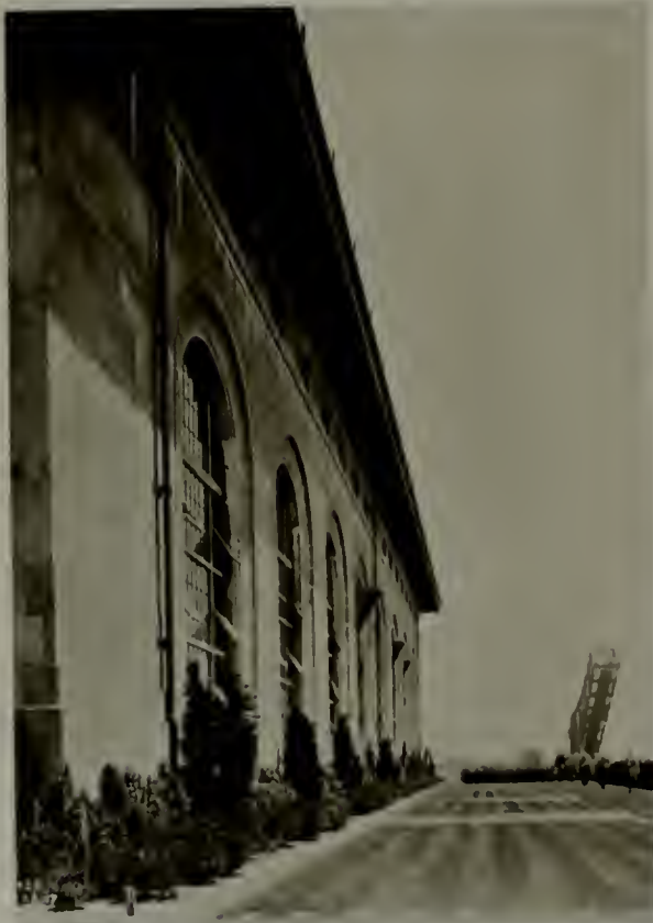
LONG BEACH STEAM PLANT
