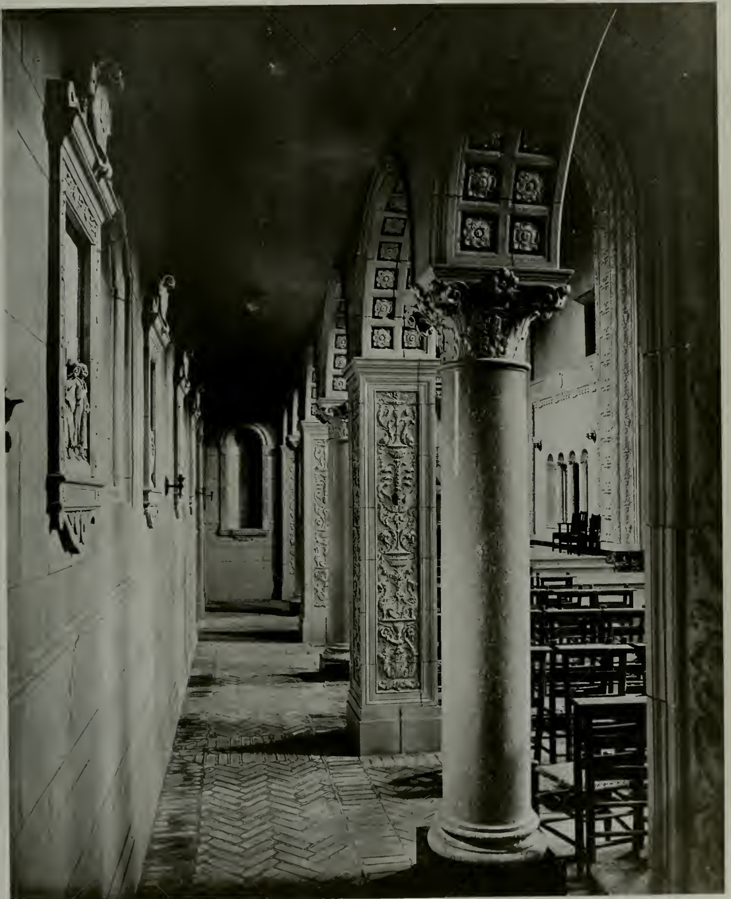
AISLE IN CHAPEL CARMELITE MONASTERY, SANTA CLARA, CAL MAGINNIS & WALSH, Architects
