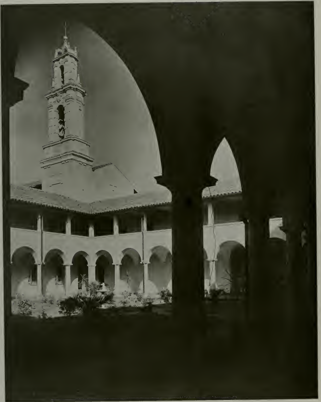
BELFRY FROM CLOISTER CARMELITE MONASTERY, SANTA CLARA, CALIF. MAGINNIS & WALSH, Architects
