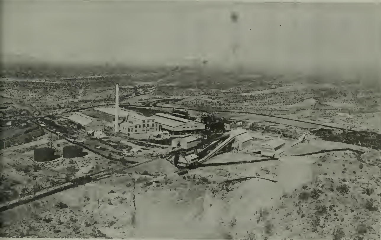
GENERAL VIEW OF PLANT
