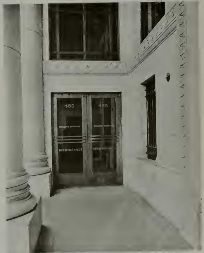
DETAIL OF ENTRANCE TO OFFICE BUILDING
