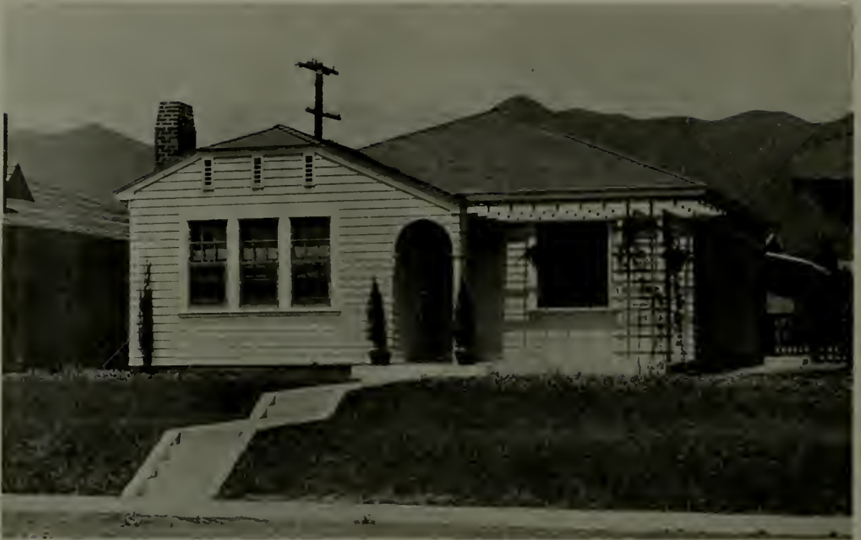
B.—THERE IS DECIDED MERIT TO THIS SIMPLE DESIGN, BUT THE SLENDER POST SUPPORTING THE ARCH APPEARS INADEQUATE
