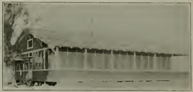
FIG. 4. THE NEW BUNK HOUSE. TWO MEN OCCUPY ONE ROOM, WITH SLEEPING PORCH
