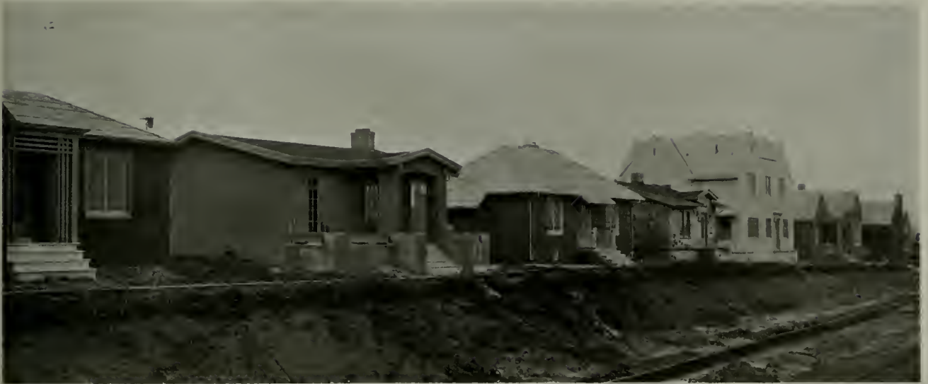
VIEW ON NORMAN AVENUE, TOWARD SUSSEX STREET, CLYDE, CALIFORNIA
