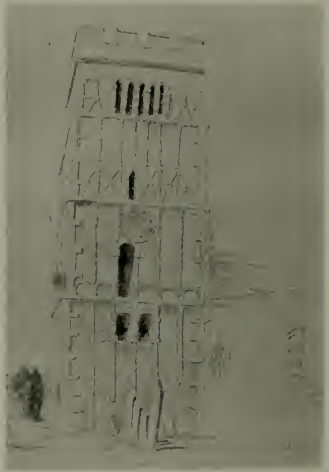
TOWER, EARL'S BARTON CHURCH **
