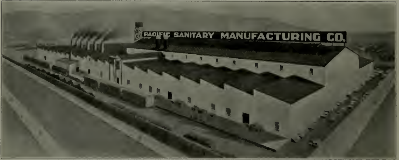
MAIN PLANT AT RICHMOND, CALIFORNIA
