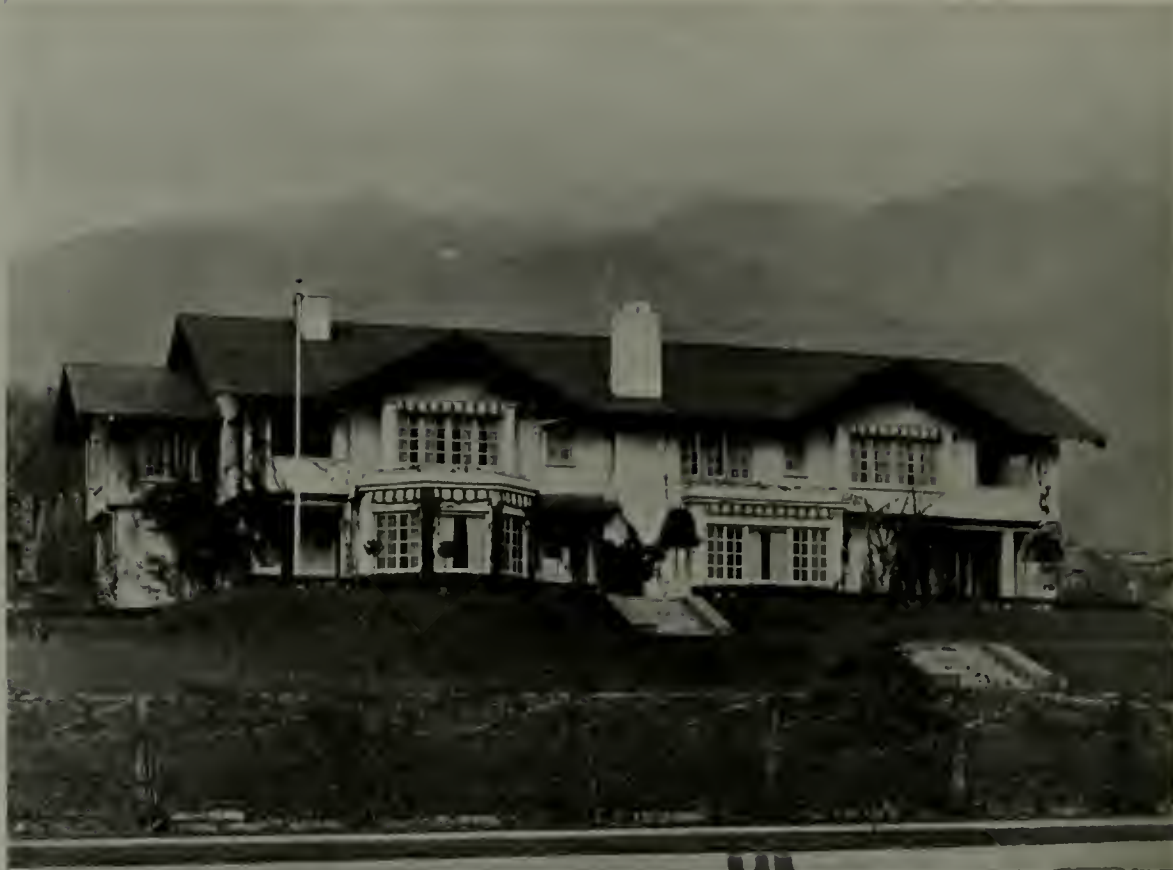
B.—THE LONG HORIZONTAL LINES WHICH GIVE CHARACTER TO THE HOUSE ARE ACCENTED BY SILLS, HEADS AND MUNTINS OF THE WINDOW GROUPS AND BY OVERHANGING SECOND STORY
