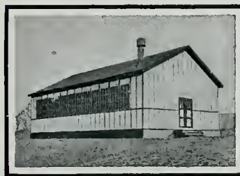
ONE STORY MILL BUILDING
