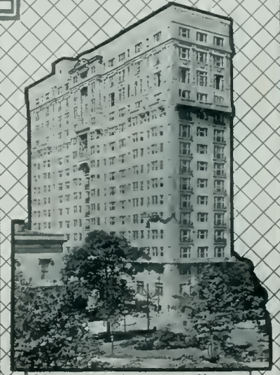
WELLINGTON APARTMENT HOTEL, PHILADELPHIA. LOUIS WANNER, PLUMBER - FRED. WEDDER, ARCHT.
