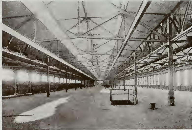
NEWEST TYPE OF SHED. INTERIOR TYPES OF HARBOR SHED. MONTREAL
