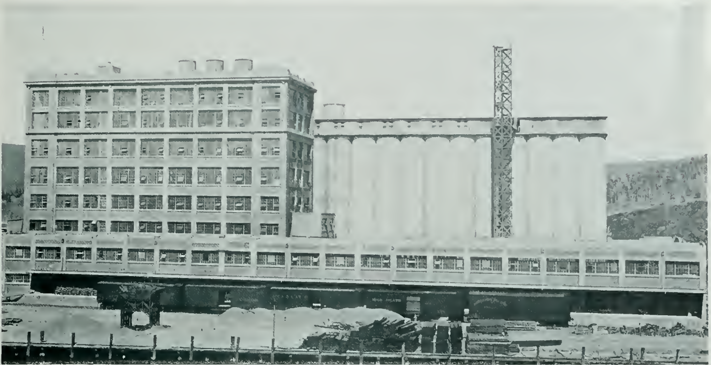
MILL AND WAREHOUSE FOR THE SPERRY FLOUR CO., VALLEJO, CAL. MAURICE C. COUCHOT, Consulting Engineer
