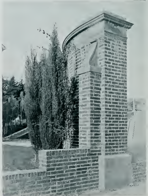
DETAIL OF GATE
