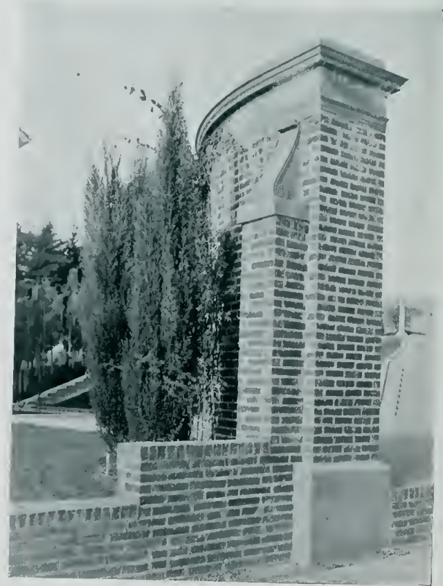
DETAIL OF GATE
