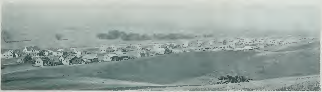
GENERAL VIEW OF CLYDE UNDER CONSTRUCTION
