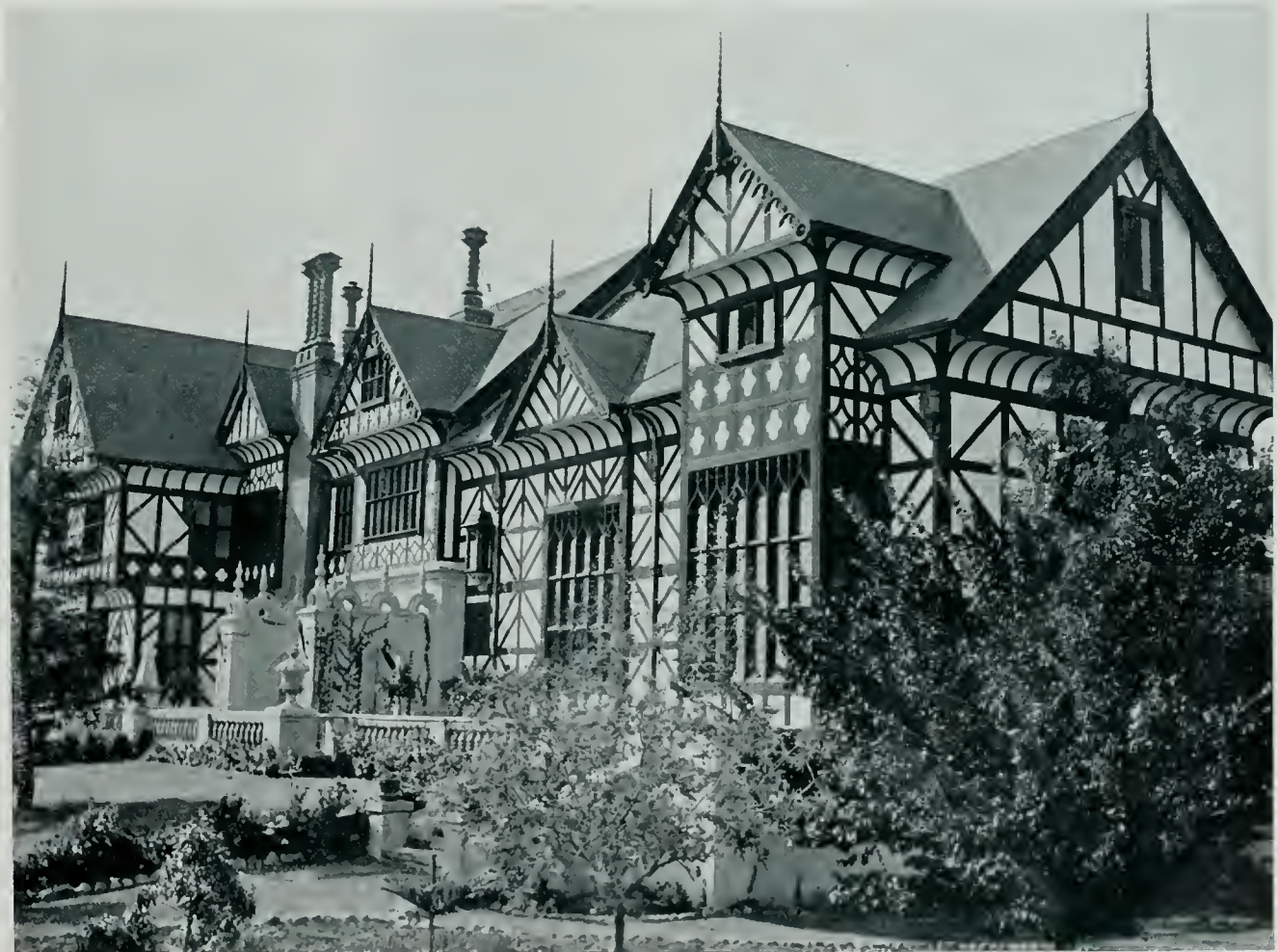
DETAIL OF NORTH FRONT
