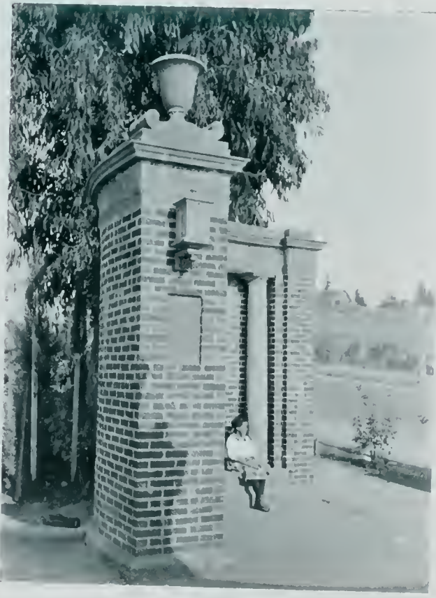
DETAIL OF GATE
