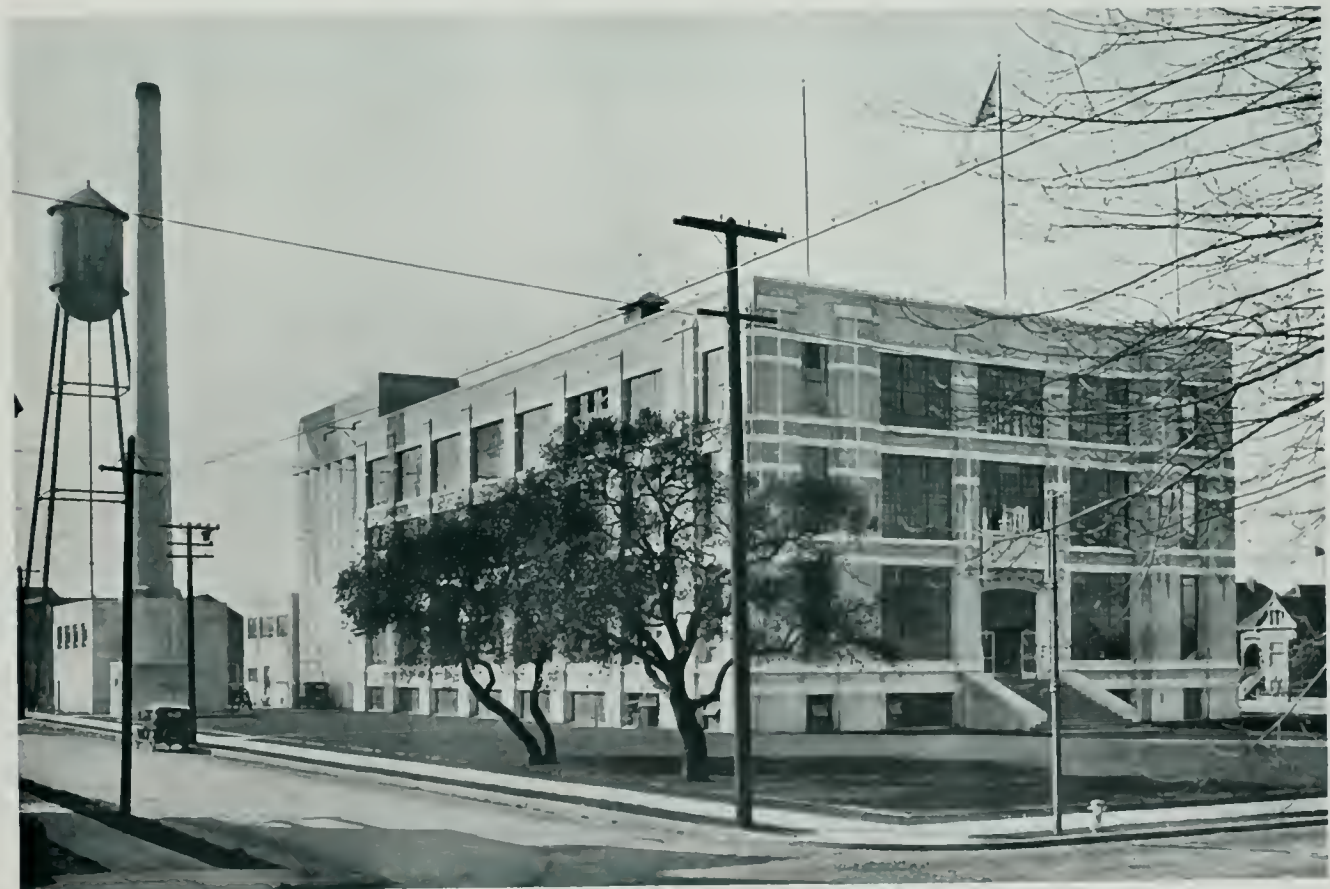
BUILDING FOR THE PACIFIC COAST SHREDDED WHEAT CO., OAKLAND, CAL. LEWIS P. HOBART, Architect CHARLES H. CHENEY, Associate
