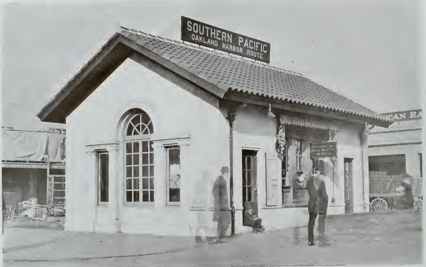
OAKLAND HARBOR FERRY TICKET OFFICE BOARD OF STATE HARBOR COMMISSIONERS, STATE DEPARTMENT OF ENGINEERING, Architects
