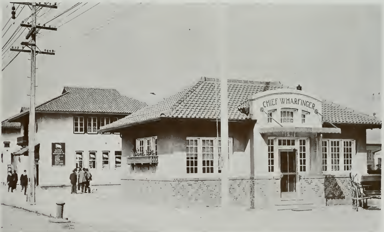
CHIEF WHARFINGER'S OFFICE AND BUILDING OF CALIFORNIA NAVIGATION AND IMPROVEMENT COMPANY STATE ARCHITECT SAN FRANCISCO WATER FRONT
