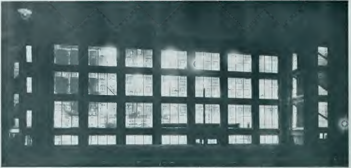
NIGHT VIEW—PLANT OF THE PACIFIC COAST SHREDDED WHEAT CO., OAKLAND, CAL. LEWIS P. HOBART, Architect. CHARLES H. CHENEY, Associate
