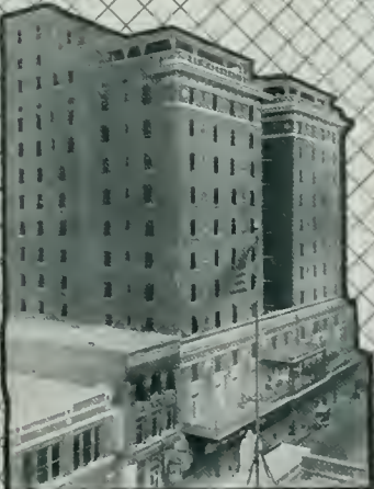
ADOLPHUS HOTEL ANNEX DALLAS THE HAMILTON CO. PLUMBERS. LANG & MITCHELL ARCHT.
