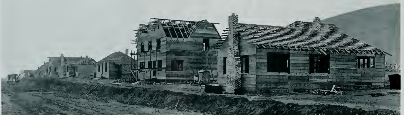
CONSTRUCTION WORK AT CLYDE
