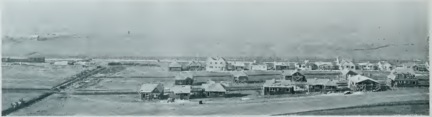
GENERAL VIEW OF CLYDE UNDER CONSTRUCTION
