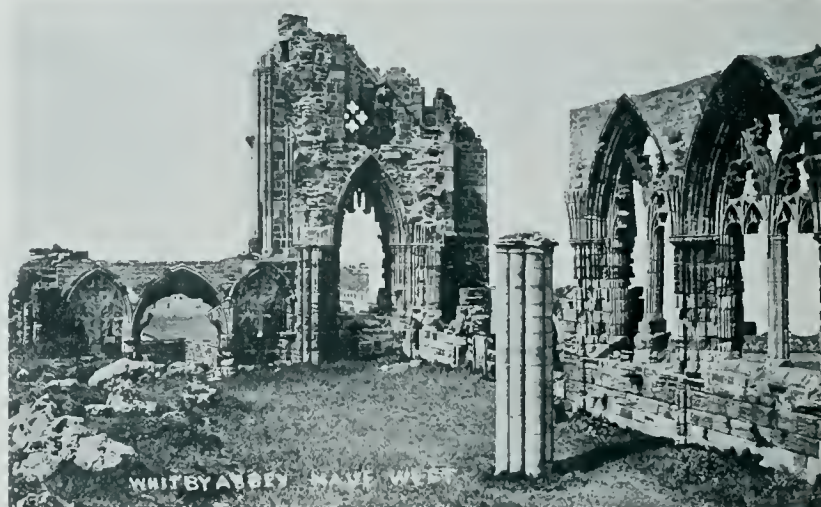
WEST NAVE OF THE ABBEY WHITBY
