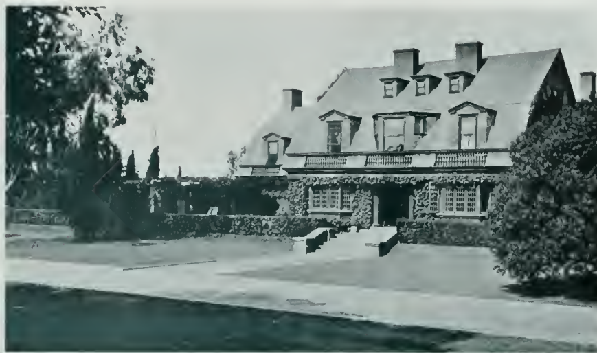
RESIDENCE OF GEORGE H. BIXBY, RANCHO "LOS CERRITOS" NEAR LONG BEACH SOUTHERN CALIFORNIA COXHEAD & COXHEAD Architects, San Francisco
