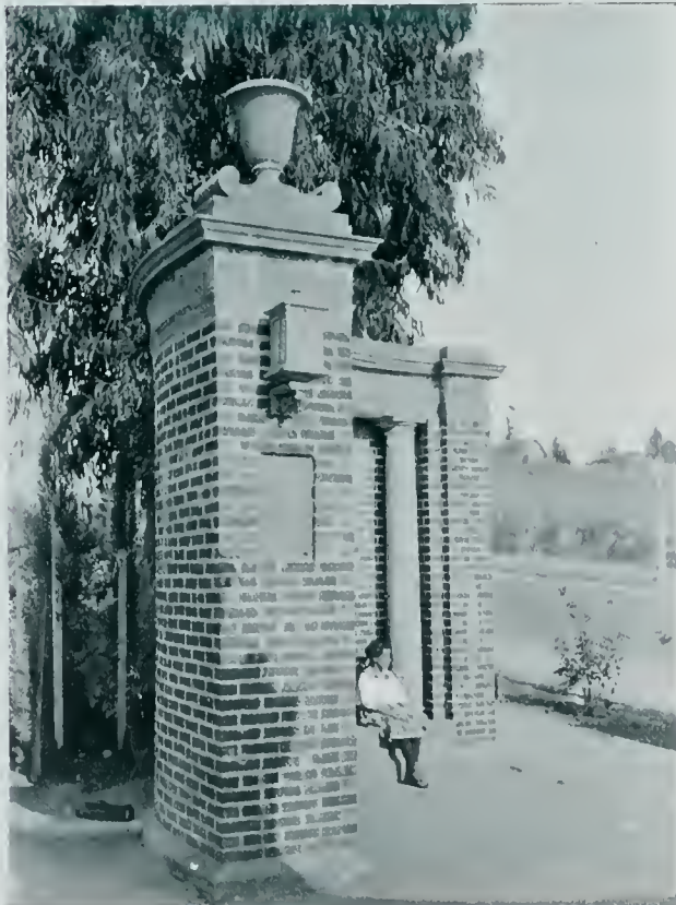
DETAIL OF GATE
