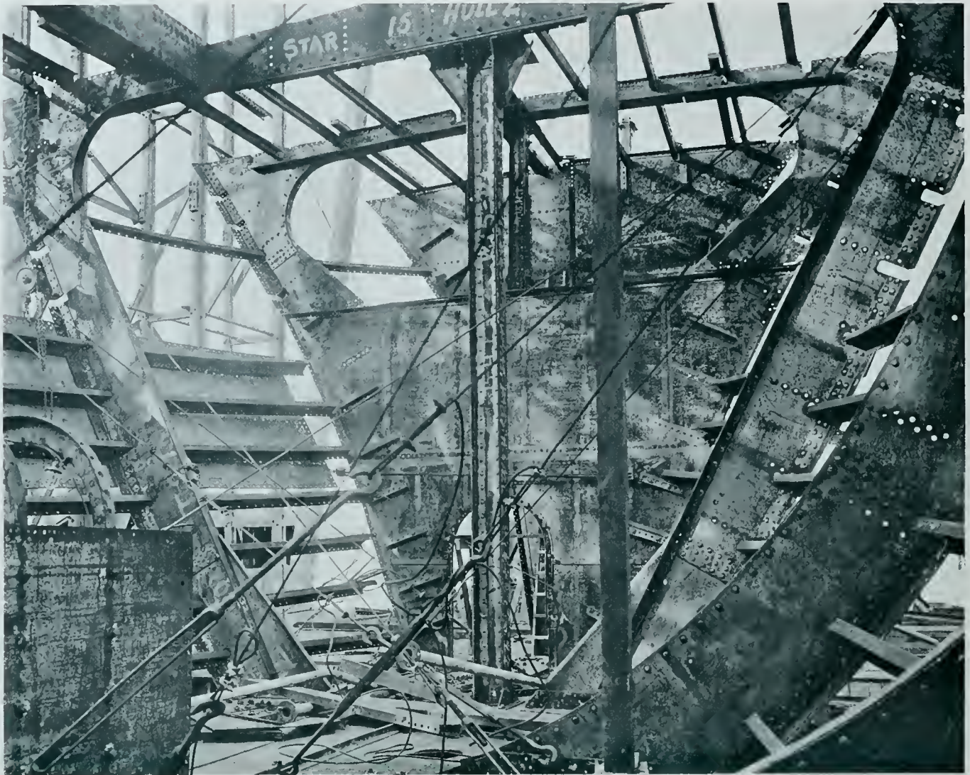
RIBS OF A 9400 TON CARGO BOAT. YARD OF THE PACIFIC COAST SHIPBUILDING COMPANY
