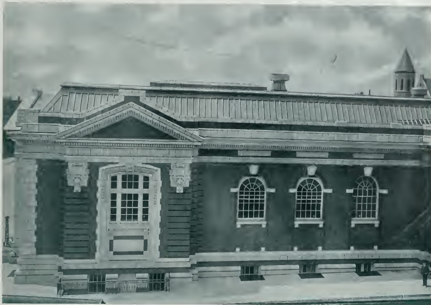
The Carnegie Library, at Frankford, Philadelphia. The tin has been laid over half-round strips to give the desired ribbed effect.
