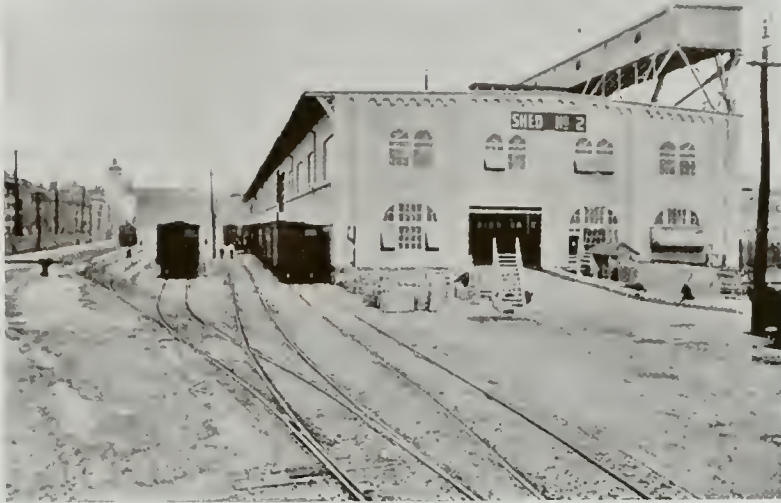
SHED NO. 2. EXTERIOR
