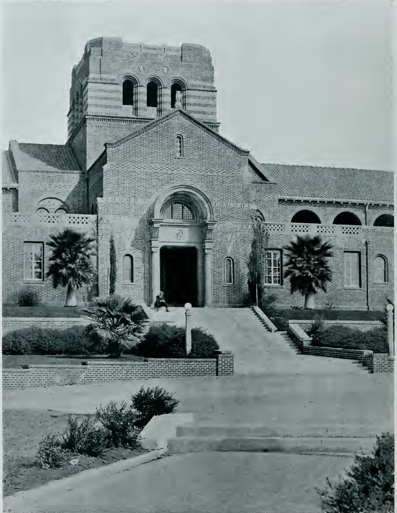
ENTRANCE DETAIL, SANTA MONICA HIGH SCHOOL, SANTA MONICA, CAL.
