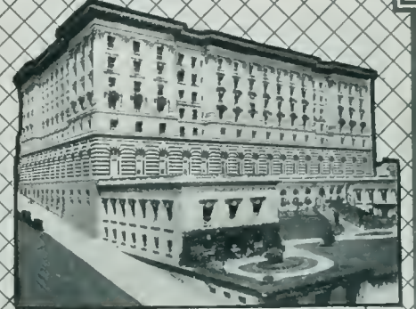
FAIRMONT HOTEL, SAN FRANCISCO. DUFFY BROS. PLUMBERS - REID BROS. ARCHITECTS
