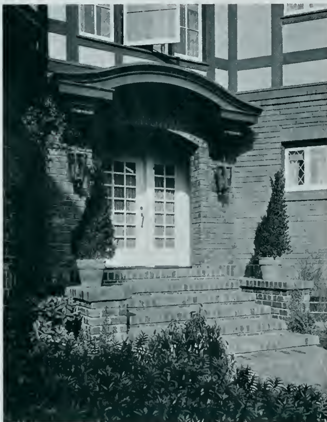
DOORWAY FOR RESIDENCE OF MRS. F. L. NELSON, OAKLAND CHESTER H. MILLER, Architect
