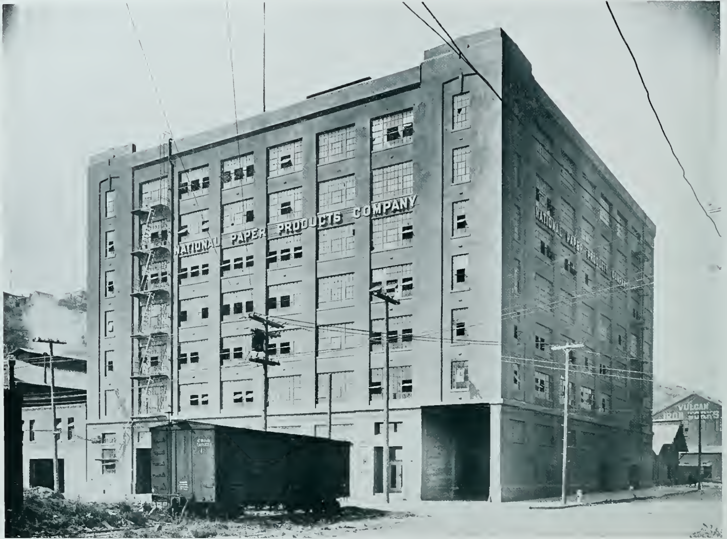
BUILDING FOR THE NATIONAL PAPER PRODUCTS CO., SAN FRANCISCO (ZELLERBACH PAPER WAREHOUSE) MACDONALD & KAHN Industrial Engineers
