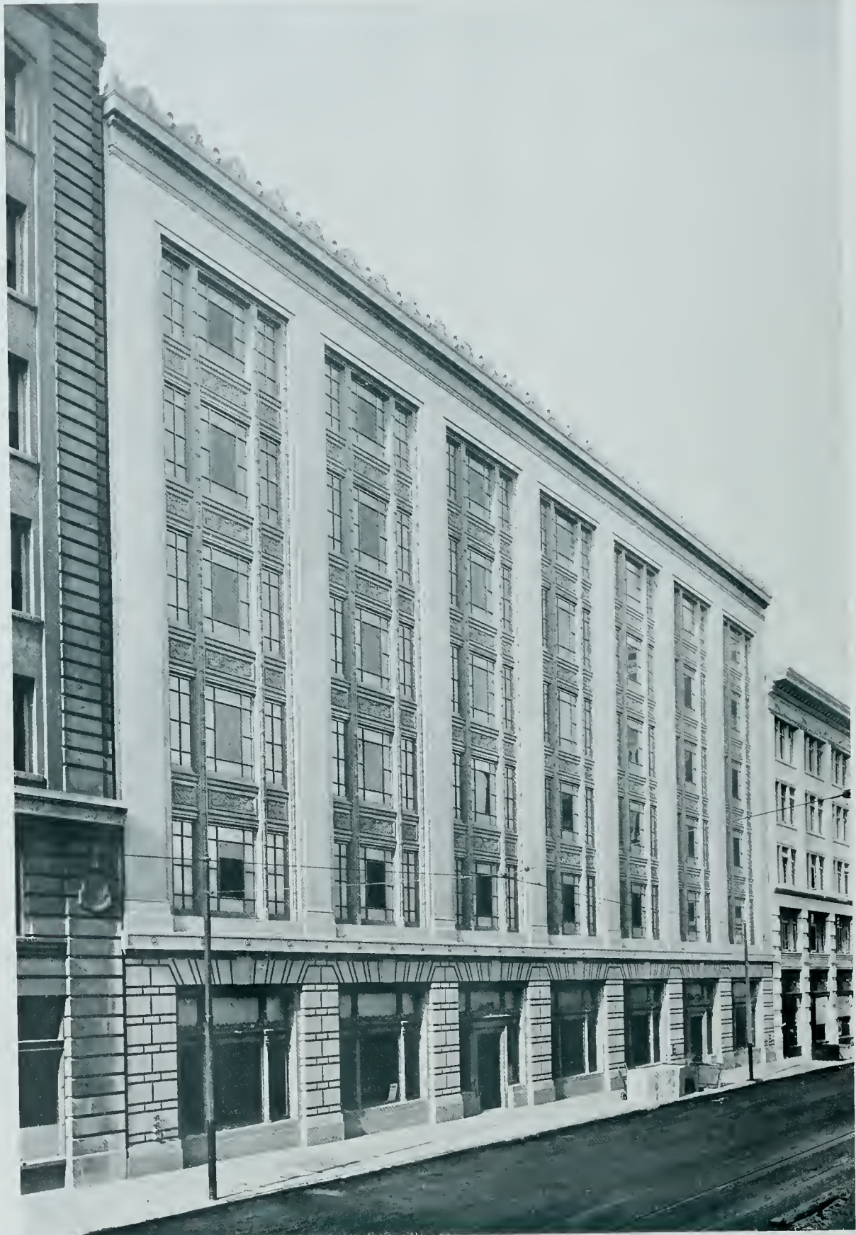
BATTERY BUILDING FOR JOHN A. HOOPER, SAN FRANCISCO KENNETH MAC DONALD, JR., Architect and Manager of Construction
