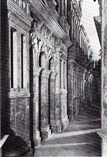
22 Part of the stage set for the Teatro Olimpico. The set with its five radial avenues leading into perspectively exaggerated depth was designed by Vincenzo Scamozzi in 1584 as a Tragic Scene in the tradition of Peruzzi (fig. 14) and Serlio (fig. 12), but realized at a monumental scale for the performance of Sophocles' Oedipus Rex in 1585 (see fig. 18).
