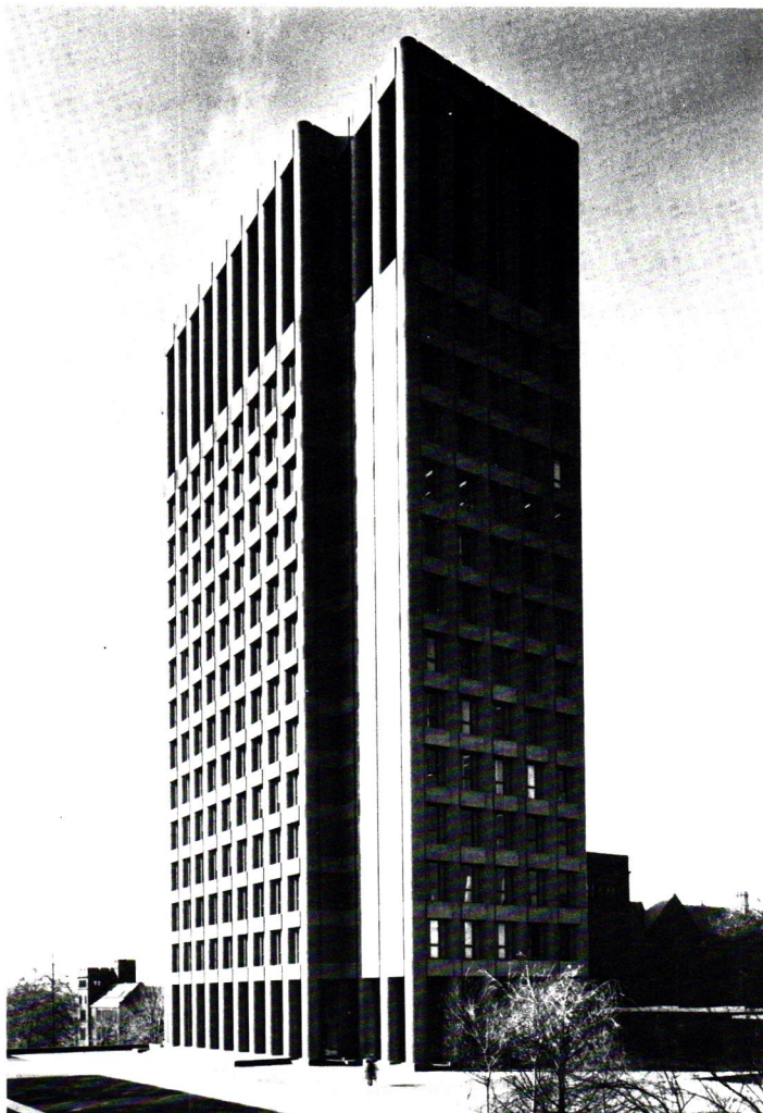
2 Kline Science Center, New Haven, Connecticut. Philip Johnson and Richard Foster, architects, 1965.
