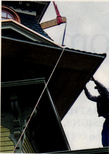
RIGHT: In a breathtaking move, the 5,000-pound roof, suspended by its lifting arms from a crane, is hefted into position atop the tower.
