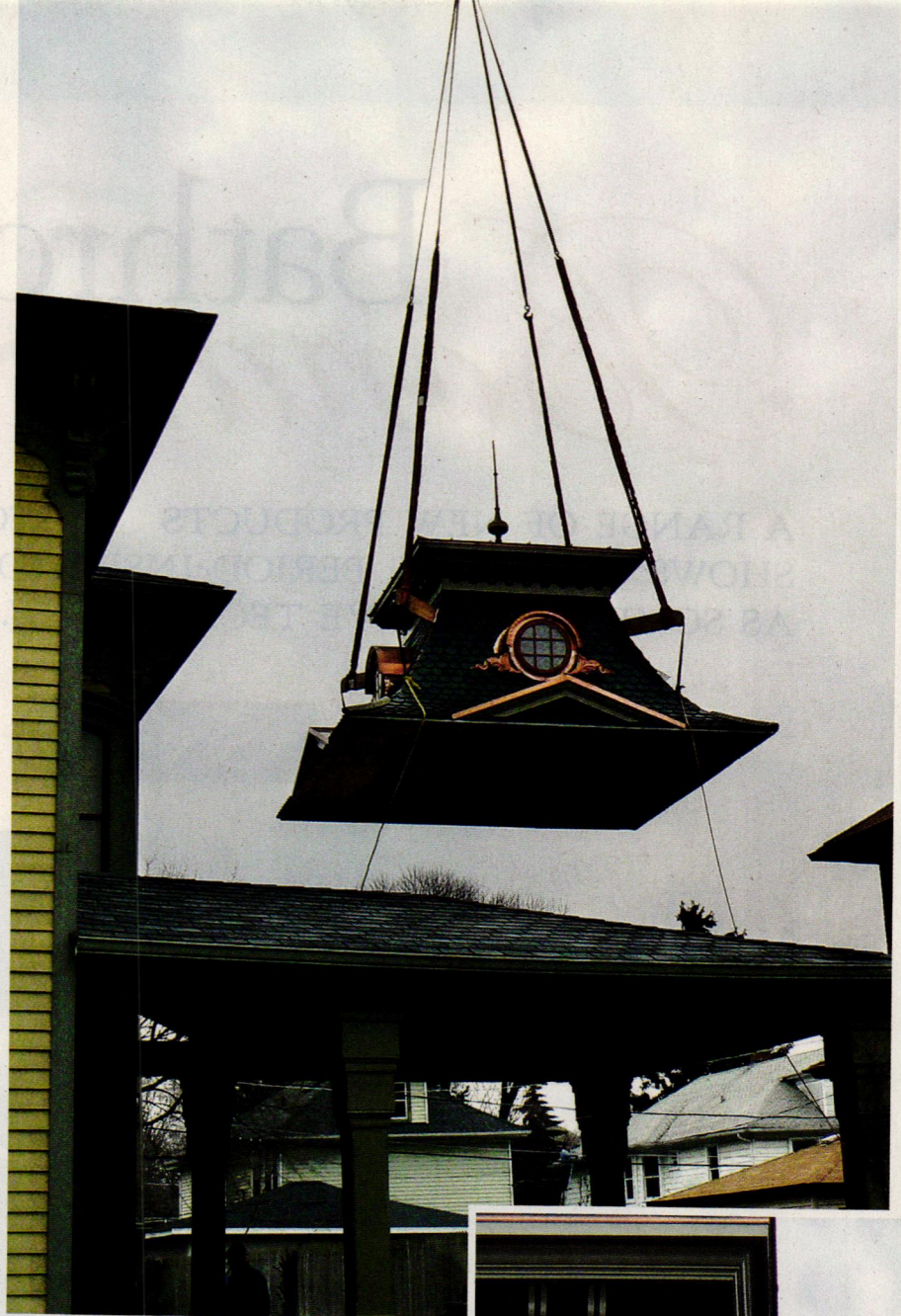
RIGHT: In a breathtaking move, the 5,000-pound roof, suspended by its lifting arms from a crane, is hefted into position atop the tower.
