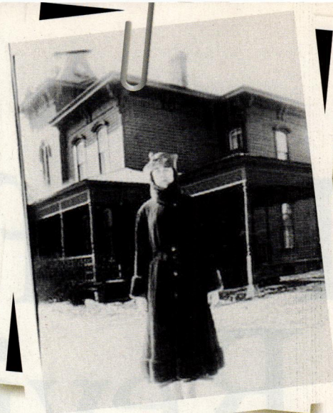
ABOVE: A 1930s photo, given to Harry by the previous owners, shows the original roof as well as early porch additions that were removed in the '50s.
