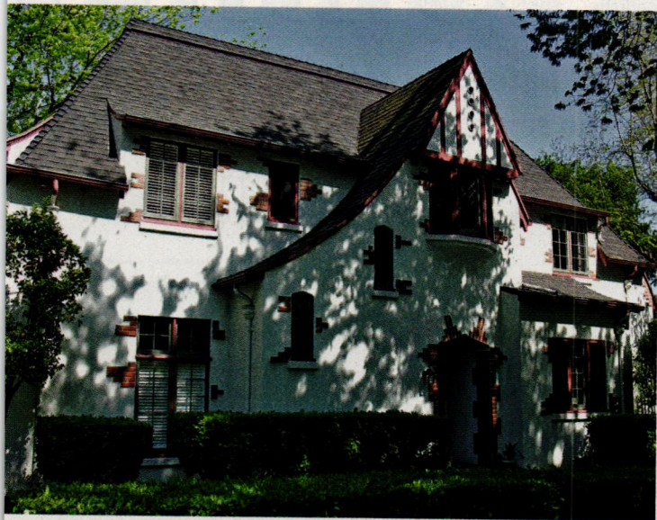
A 1927 house with a dramatic catslide gable around the front door, topped by a gem of a diamond-paned oriel window, shows extensive Old English characteristics. The steep hipped roof, and the brick accents around casement windows, could appear as easily on a Norman house as on an English one.
