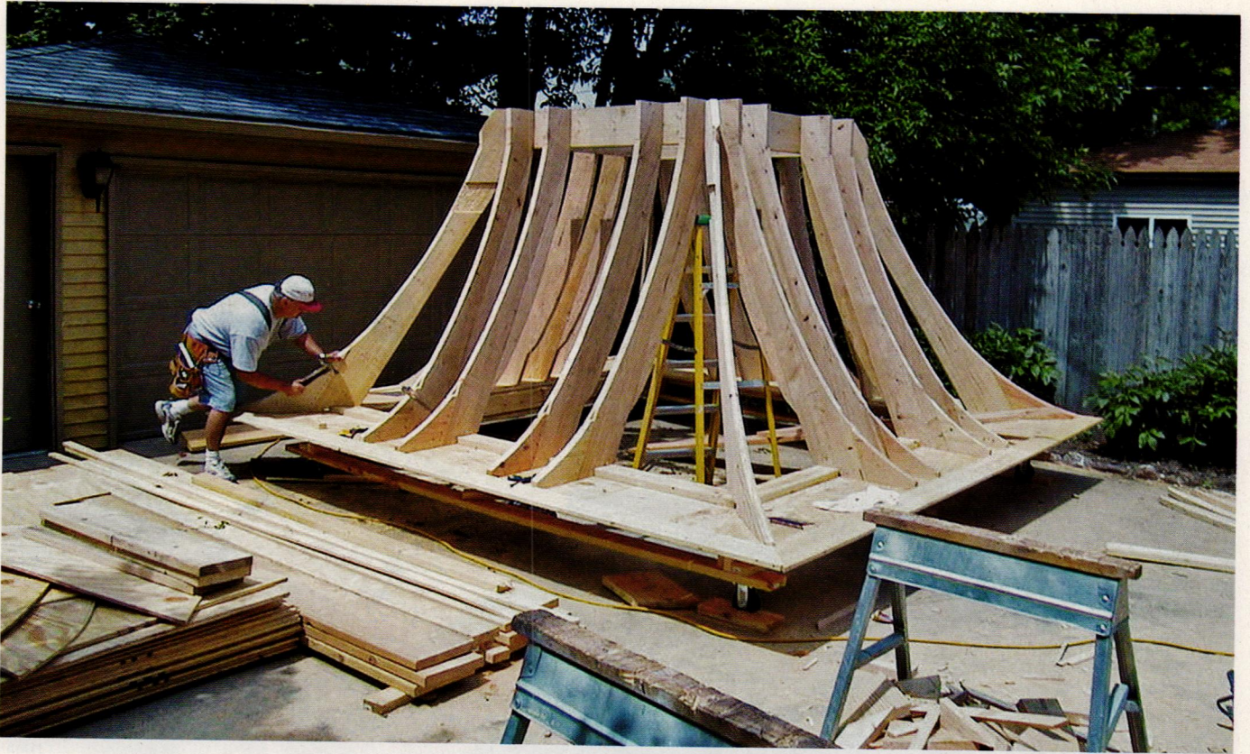
Working on the ground in Harry's driveway, Rich first assembled the ribs, which he cut using a template and a heavy-duty jigsaw.
