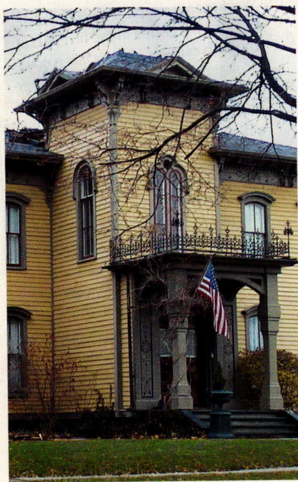
ABOVE: A view of the truncated tower before restoration. "It just didn't look right," says Harry. "You could tell something was missing."
