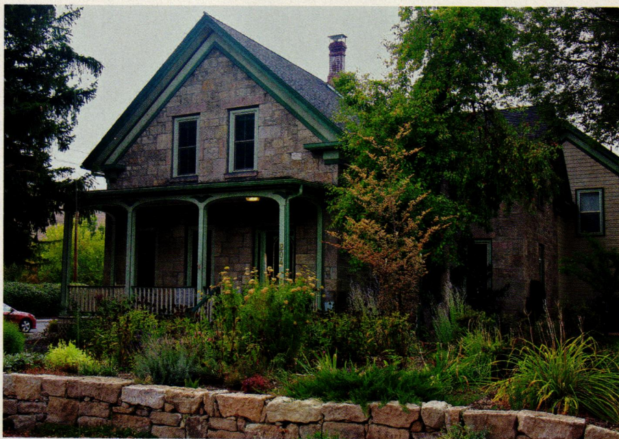
TOP: No fewer than three bay windows adorn the 1875 Olcovich-Meyers House, designed in a late Italianate style with Gothic Revival gables. ABOVE: The warm-toned local sandstone is used in major public buildings and in a few houses, including the circa 1883 Edwards House, where it was laid in a random ashlar pattern.
