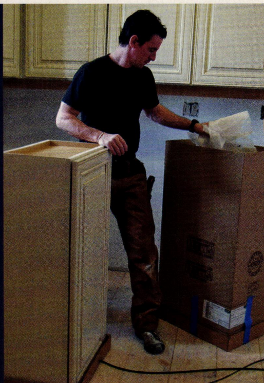
ABOVE: It's important to ensure that the cabinets are level and plumb in all directions. To guarantee that this is the case, Mark carefully checks all of the surfaces using a torpedo, a 2' level, and a 4' level consecutively. Then he double-checks it.
