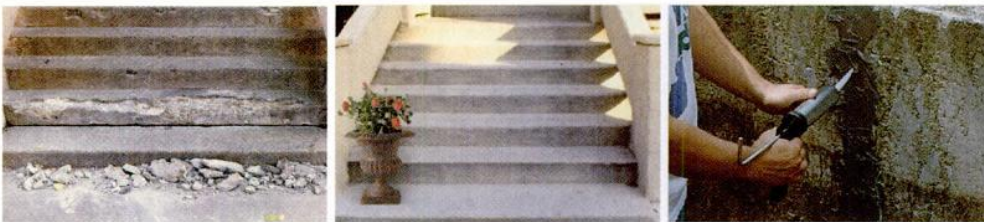
Abocrete can be used to replace missing concrete.
