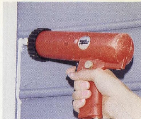
Use of an air regulator on the compressor or the line is highly recommended for pneumatic caulking. Too much pressure can be explosive.
