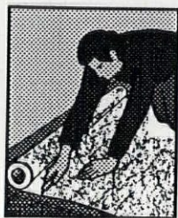
1. Cut fiberglass mat 2" longer than height.
