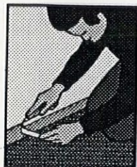
5. Trim mat at baseboard and window.
