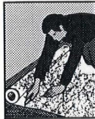
1. Cut fiberglass mat 2" longer than height.
