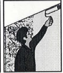
8. Apply 1st coat of saturant to adjacent area.
