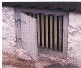
Paint changes as it ages. Most common is yellowing of linseed-oil binders when hidden from light.
