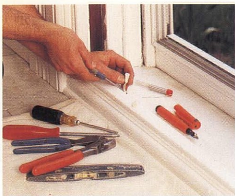
All devices should be hermetically sealed and wire connections should be soldered.
