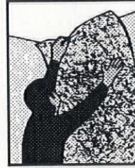
3. Apply fiberglass mat to wet surface.
