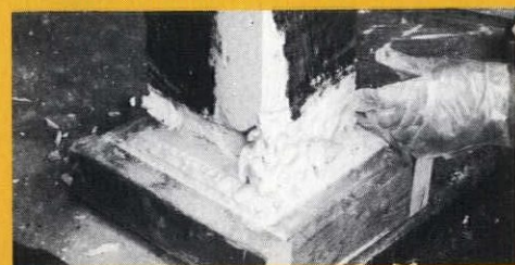
...were completely sawed off and replaced with...
