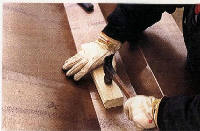
Once the bends are interlocked, flatten them down to crimp the seam and to prevent a ridge in the gutter.
