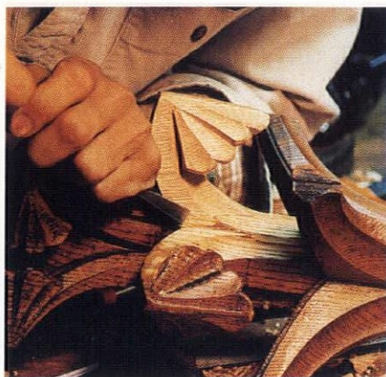
After the epoxy is cured, repaired necks are trimmed back to the lines of the original ornament.
