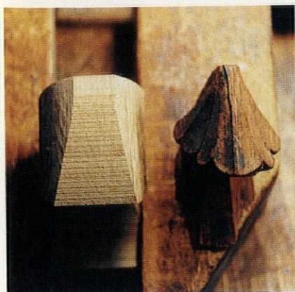
To repair this finial knob, David Calvo first saws out a block of wood as close in shape as possible to the original.
