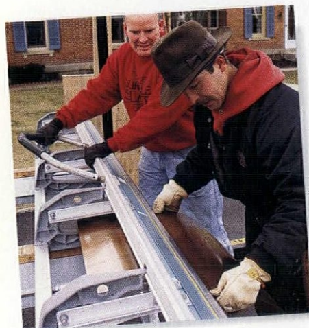
ABOVE: The metal must be bent to shape, a process that's made easier with the use of a bending break. BELOW: Draw solder into the seam by placing the iron directly over it.
