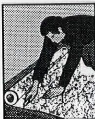
1. Cut fiberglass mat 2" longer than height.
