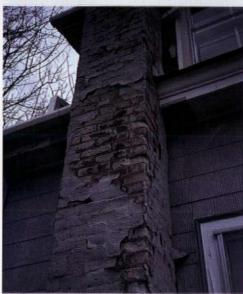
TOP: Creosote on the exterior of the chimney means big problems: condensation, interior creosote buildup, and deteriorated masonry. ABOVE: Sometimes soft brick was used to build chimneys. This masonry does not stand up well to flue gases or weathering.
