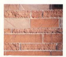
TOP: Although less commonly built, some sandstone houses, such as this 19th-century example, were two storeys high with Greek Revival embellishments. ABOVE: Slab-and-binder masonry alternated face-cut and bed-cut sandstone.
