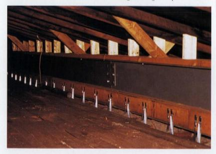
were bolted together, they formed two 35' beams that ran the length of the attic.
