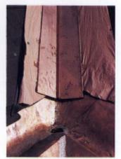
FAR LEFT: Cleats provide anchors without penetration and give the metal freedom to move. MIDDLE: If you're replacing flashing on an existing roof, you'll need to remove adjacent roofing. LEFT: The bottom edge should be doubled under and formed into the gutter system.
