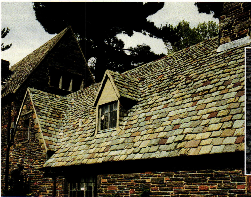
LEFT: Graduated roofs reduce the slate thickness as the courses approach the ridge. BELOW: Slates over 1" at the butt often begin the graduated roof.
