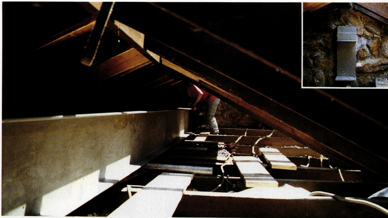
TOP PHOTO: Pipes made quick work of rolling the 30’ steel beam into the kitchen attic. A wood beam would have been impractical in this confined space. INSET: Behind the custom-fabricated plate is a horizontal shelf cut and grouted into the massive chimney so that it can support the steel.
