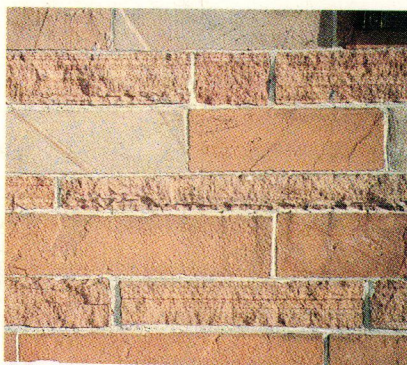
TOP: Although less commonly built, some sandstone houses, such as this 19th-century example, were two storeys high with Greek Revival embellishments. ABOVE: Slab-and-binder masonry alternated face-cut and bed-cut sandstone.
