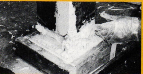
...were completely sawed off and replaced with...
