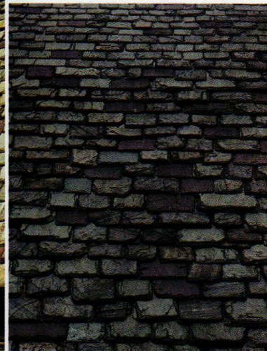
LEFT: Graduated roofs reduce the slate thickness as the courses approach the ridge. BELOW: Slates over 1" at the butt often begin the graduated roof.
