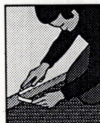
5. Trim mat at baseboard and window.
