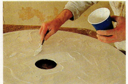
Make sure to get a good, thick coat of adhesive on the back of the run surround.
