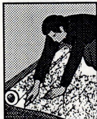
1. Cut fiberglass mat 2" longer than height.
