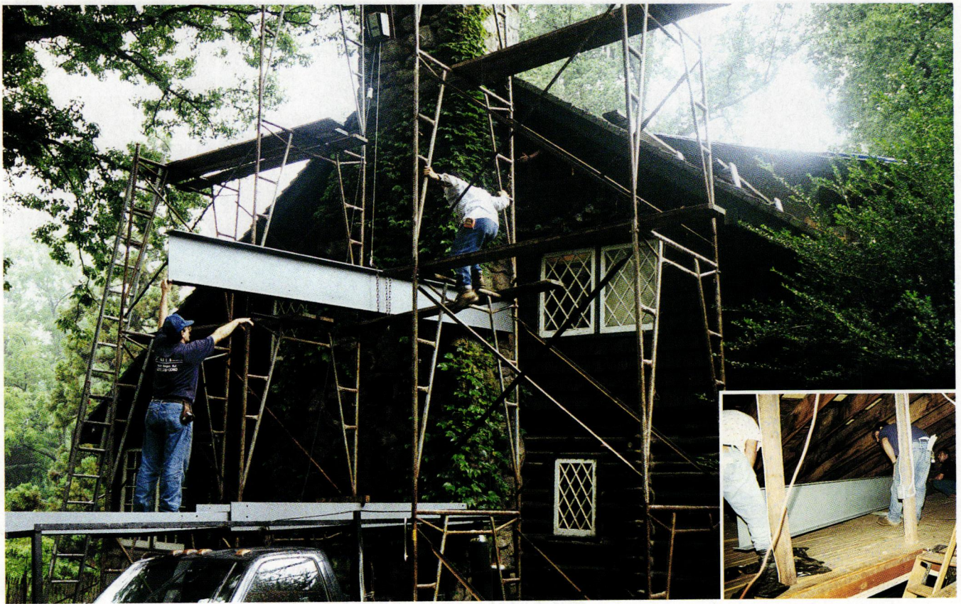
ABOVE: An attic vent window (above worker in photo) provides a way into the main building for the dormer steel. INSET: More pipes position the steel once inside. BELOW: Now in place, one two-piece dormer beam is connected to the existing framing by cripples and fasteners.
