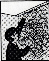
4. Trim excess mat where wall meets ceiling.
