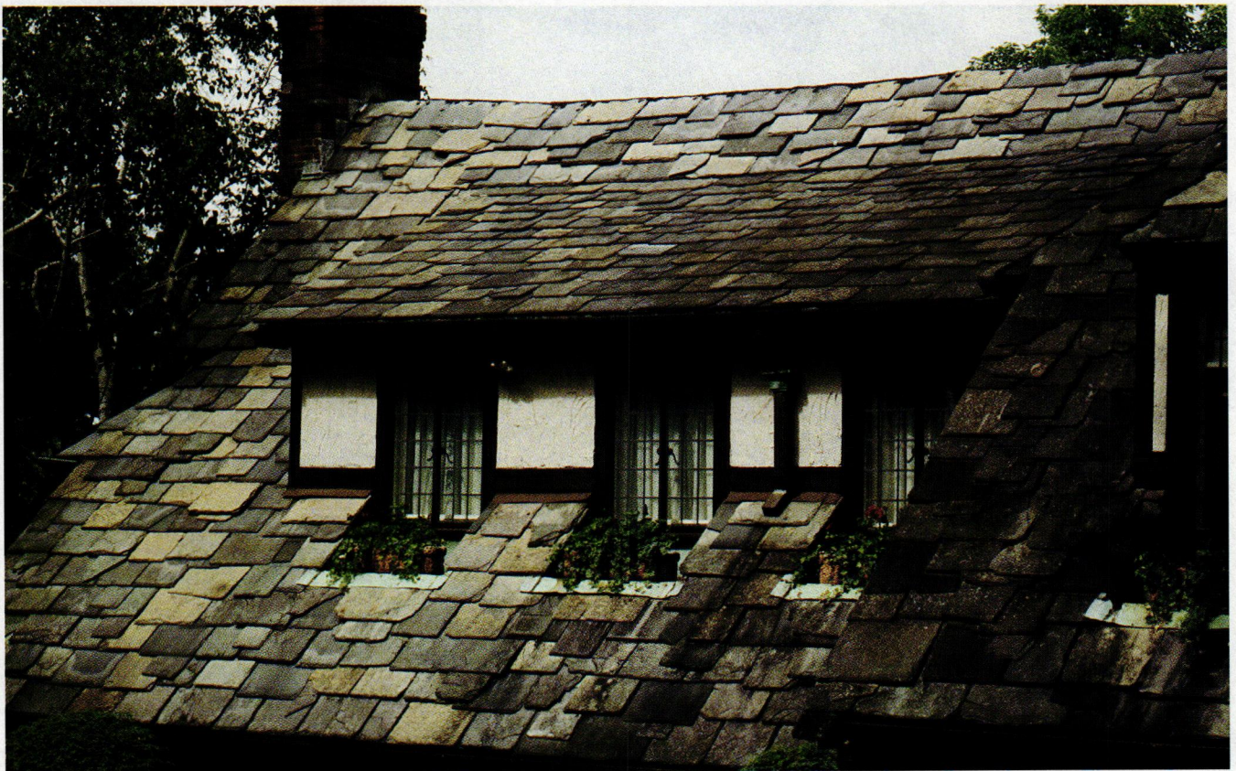
Textural roofs scramble slate thicknesses, lengths, widths, and colors in combinations that can be specified for any one of many rustic looks. The effect is most often seen on average slopes; steep roofs and towers tend to look “cut up.”
