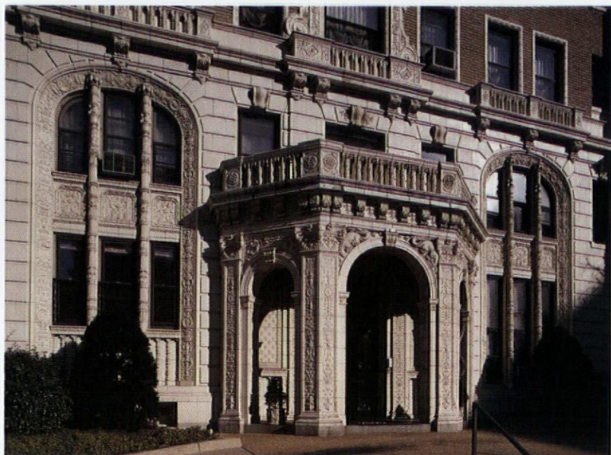
Many of the best apartment houses were identified only by address, rather than by pretentious names. A major feature of fashionable apartment buildings was a grand entrance with an equally grand lobby inside. This terra-cotta example in Washington, D.C., is one of the finest.
