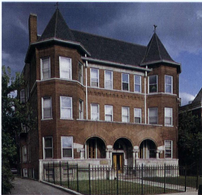
This Romanesque Revival building has an apartment on either side of a common entry, typical of many Chicago Six-Flats.
