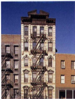
The line between New York tenements and middle class apartments can be slim, perhaps no more than a fancy broken pediment at the roof.
