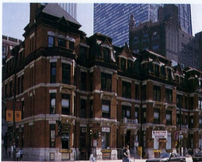
This grand early Chicago apartment building featured French flats, a term reserved for more elegant front-to-back apartments. Note the several entrances, each providing access to four or eight flats.
