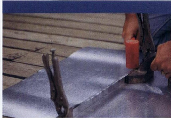
Work as far along as possible between locking pliers.
