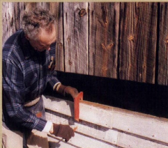
Marking along the buzzard's finger produces more accurate cuts than measuring.
