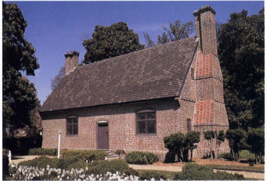
The Adam Thoroughgood House, in Virginia Beach, Virginia, was built c. 1640. Note its two massive chimneys: one inside the walls of the house and another, originally for cooking, on the outside.
