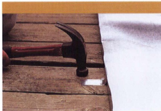
Nail the clip to the decking.
