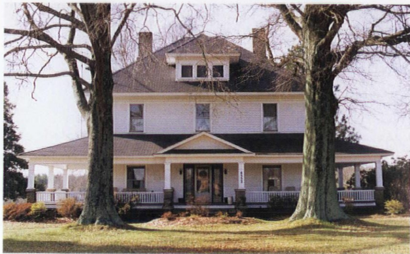
The large proportions and wrap-around verandah of the Miller house suggests the Colonial Revival style. However, its cube shape and unadorned exterior are indications of its true type — the Foursquare.
