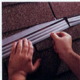
Install the Shingle Shield under a course of shingles on each side of the ridge.
