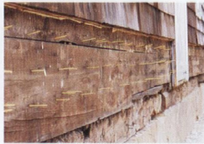
Toothpicks rendered random nail holes into the course lines characteristic of early clapboards.
