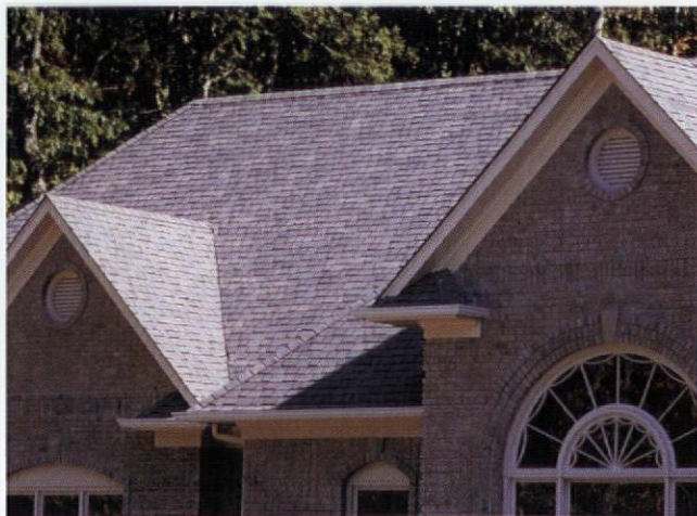
Laminated asphalt shingles build up five or more shaped layers at random to simulate the textures and shadows of natural materials.
