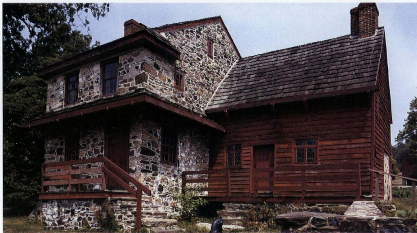
The wood frame portion on the right of the Gilpin House, in Chadd's Ford, Pennsylvania, is from 1698. The larger stone section was added in 1745.
