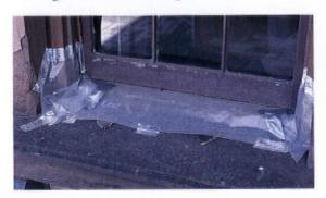
Poly sheeting keeps the sill dry and flips up for work.
