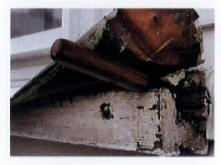
An ice pick wasn't necessary to find the decay going on under this metal-clad sill.
