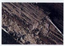
(top) Priming checks with epoxy consolidant. (middle) Working epoxy filler into checks. (bottom) Scraping away excess filler.
