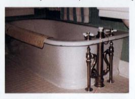
not meet modern codes. Many old tubs have the water inlet installed below the overflow outlet - an arrangement that can allow a full tub of water to backsiphon into the inlet. This creates a potential for contaminating the supply with waterborne bacteria, such as those responsible for hepatitis. Most states require that the inlet be two pipe diameters above the flood
