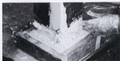
...were completely sawed off and replaced with...
