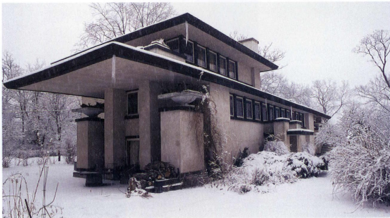
Individual panels of Prairie Plaster (above) might be finished in different color tones or combinations. With its long cantilever roof and stucco cladding, the Tomek House (below) in Riverside, Illinois, is a typical Wright Prairie building and a prototype for the famous Robie house.
