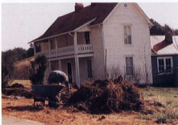
After excavating the crawl space under the house, the surplus soil was used to make the property level on the up-hill side.
