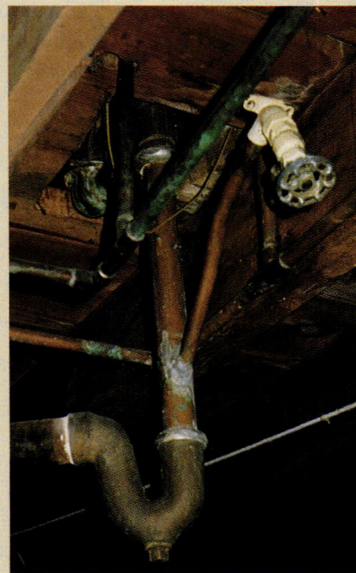
Traps often hide in awkward locations, such as this under-floor crawlspace.
