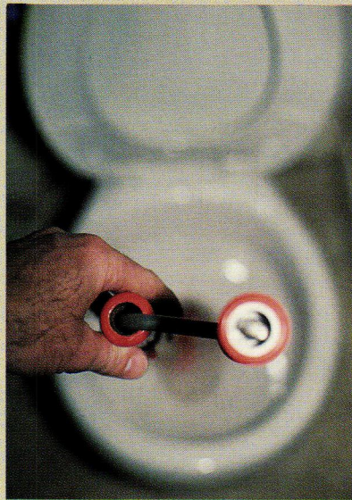
Top left: The force cup is a basic tool for tubs, sinks and toilets; closet augers are manual snakes for toilet traps. Bottom left: An electric snake, available at rental houses. Above: Closet augers are fully extended when the crank meets the shaft.
