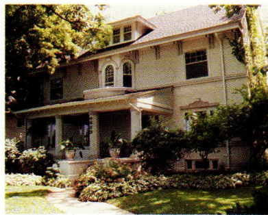
Evidence of the original Mission-style details (top) remain in this 1907 house today (above).
