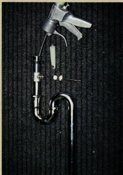
Left: When snaking a lavatory drain, begin at the outlet after first removing the stopper (which may block the snake). Right: If the snake binds at the trap, disassemble it or enter at a cleanout closer to the blockage.
