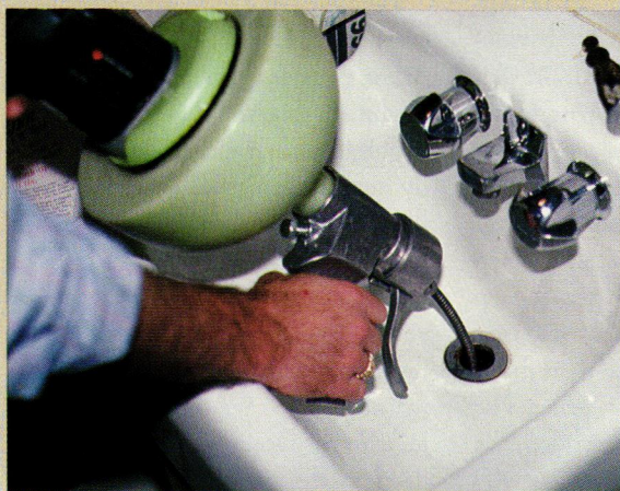
Electric snakes are cord-powered tools that should only be used if grounded and in good operating condition. Battery-powered models are also coming on the market.
