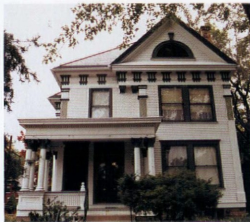
Classical porch columns used in groups key this house as a Free Classic Queen Anne.
