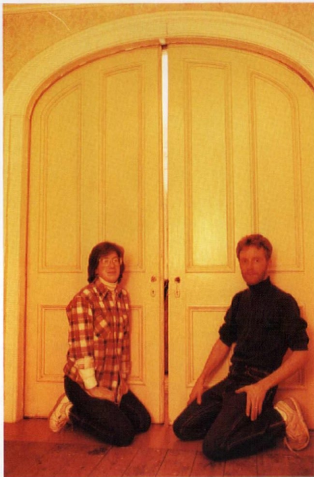
Although the sellers said that there weren't any pocket doors, Alan and I discovered this pair during the restoration. Two more sets were found in the other apartments upstairs.
