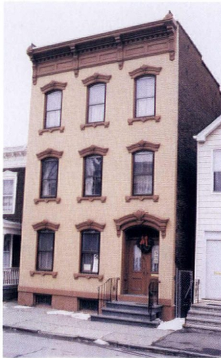
The installation of new front railings and gutters are some of the countless jobs we completed.
