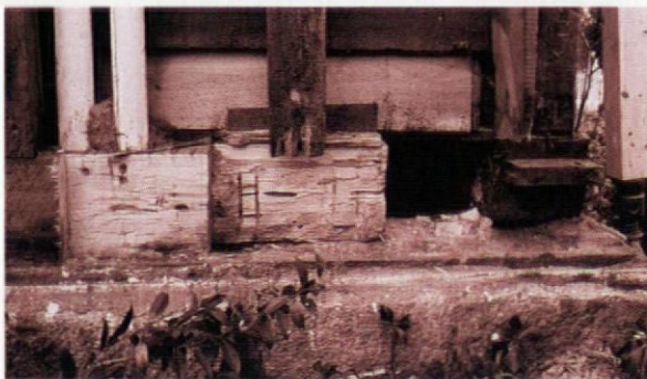
Built-up plank sill repair: After removing the decay (above), Bill squared-up the end of the existing sill with a hammer and chisel. The cleaned-up sill is cut back in steps (below) so that the new lumber is spliced in for maximum integrity.
