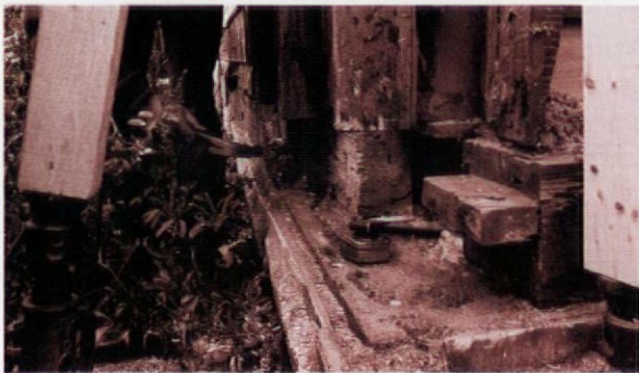
Built-up plank sill repair: After removing the decay (above), Bill squared-up the end of the existing sill with a hammer and chisel. The cleaned-up sill is cut back in steps (below) so that the new lumber is spliced in for maximum integrity.
