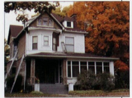
A house in Valparaiso in three stages of preparation: strip, sand, and prime.
