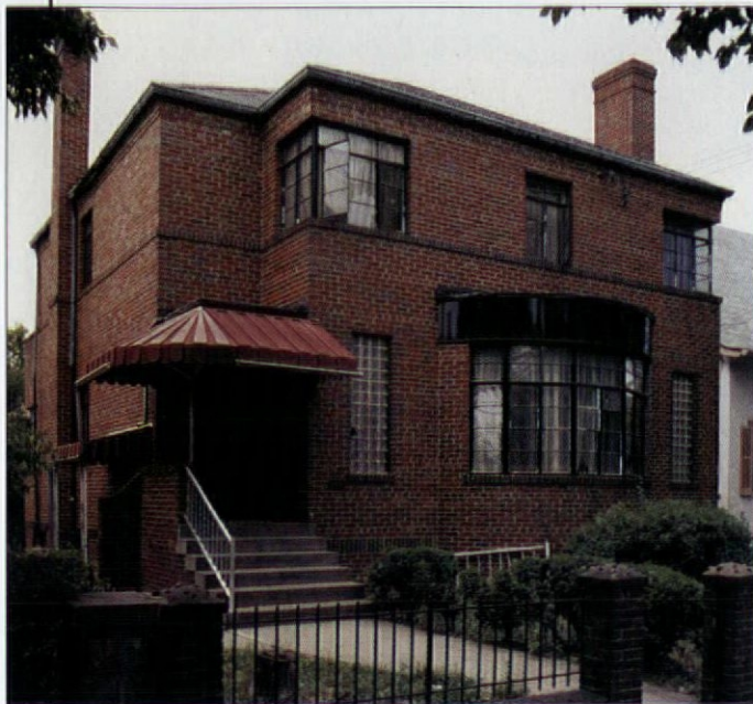
A Moderne block that catalogs window treatments of the style: bow and corner windows, steel casements, and glass block. (Washington, D.C.)
