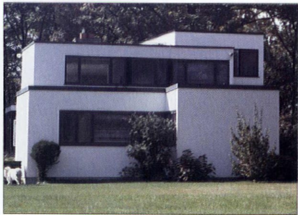
Despite its modernity, Walter Gropius' own house has a simple angular design that fits the New England tradition. (Lincoln, Mass., 1938)
