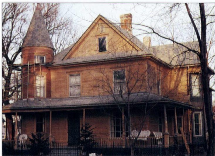
Top: My "before" photograph of the "Stormy," a dark, grey shadow of a Queen Anne. Above: Stripped and sanded, with a newly resided upper tower, the "Stormy" displays its excellent carpentry.
