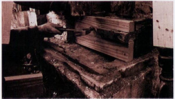
Each plank of pressure-treated lumber is fitted in and around neighboring frame parts (above). The first, second, and third planks were fastened with galvanized drywall screws (below); outer longer planks were nailed on.
