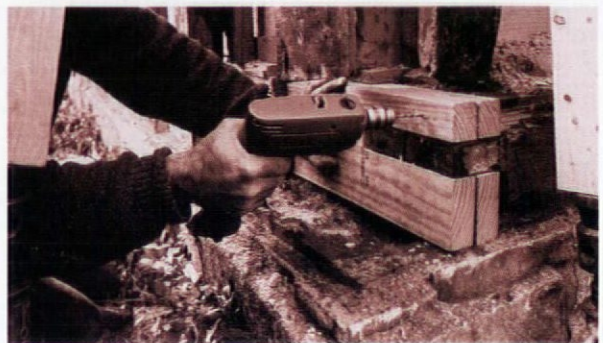
Each plank of pressure-treated lumber is fitted in and around neighboring frame parts (above). The first, second, and third planks were fastened with galvanized drywall screws (below); outer longer planks were nailed on.
