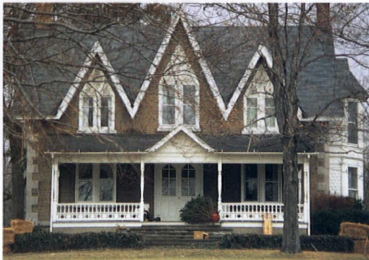
Lime mortars have time-tested durability, as evidenced by the health of this circa-1850 cobblestone Gothic Revival example.
