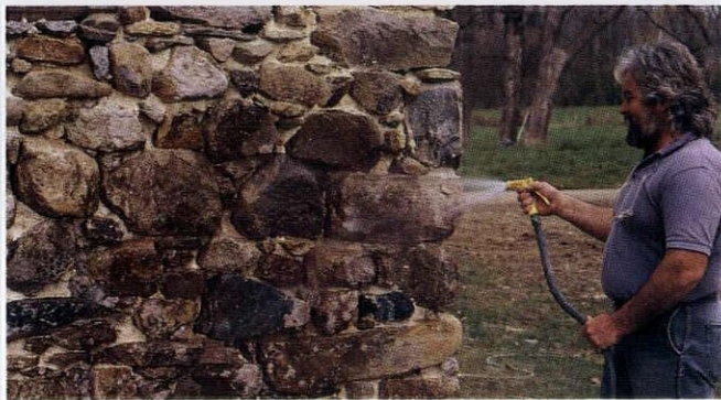
Wetting joints is important at two stages: to clean newly chipped joints, then to dampen masonry before repointing.
