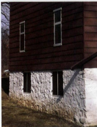
Whitewash had many historical uses, including painting simple wood buildings, fences, greenhouses, and stonework of all kinds (left). Basically a thin mix of lime and water, whitewash is applied with a wide, fiber-bristle brush (right).
