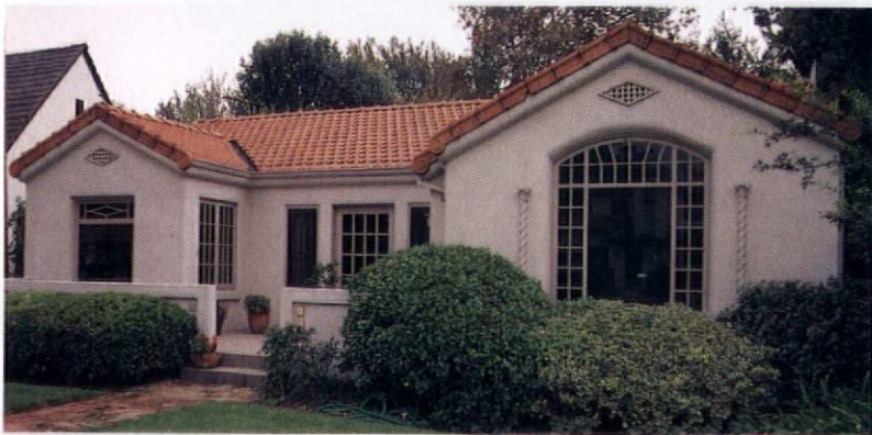
Top: The typical Spanish features of this Pasadena, California, house include false balconies with wrought-iron grilles, a classical doorway, and an arched entry to a rear yard. Middle: The roof of this Mission Style in Cape May, N.J., is shingled rather than tiled, and the scalloped gable betrays the residence's Spanish roots. Above: Projecting bays of this Claremont, California, bungalow create a Mediterranean Style, courtyard-like space.
