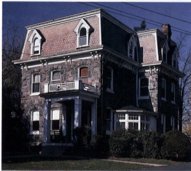
Grand Second Empire buildings were likely to be masonry like their European models, but modest houses such as this 1875 straight-roofed example are also found in stone.
