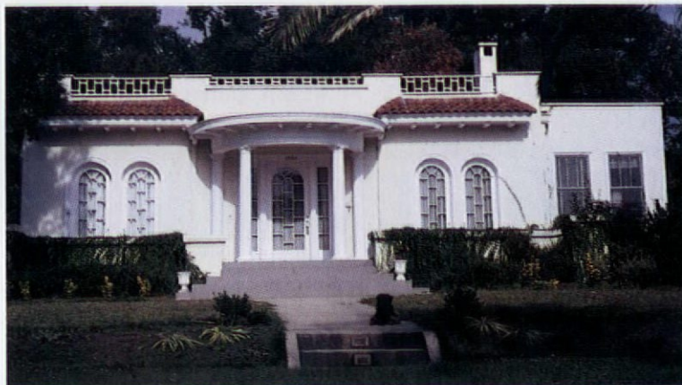
Facade symmetry and a formal entryway impart an Italian look to this circa-1910 Mediterranean Style, Pensacola, Florida, house. The main roof is flat behind the balustrade.
