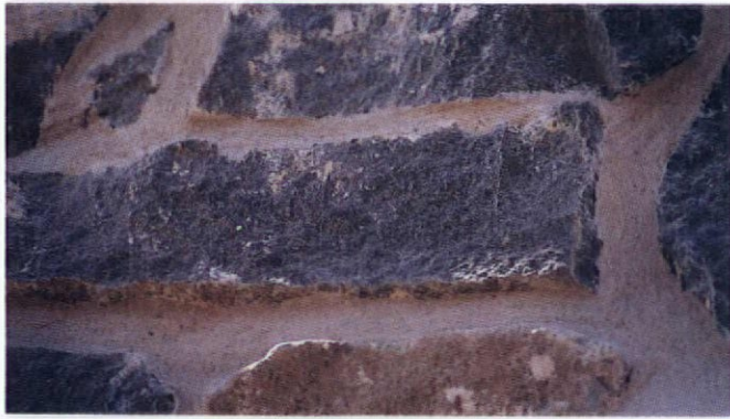
A fresh, unbrushed reveal point filled to a depth just below the stone's surface, which highlights its texture.
