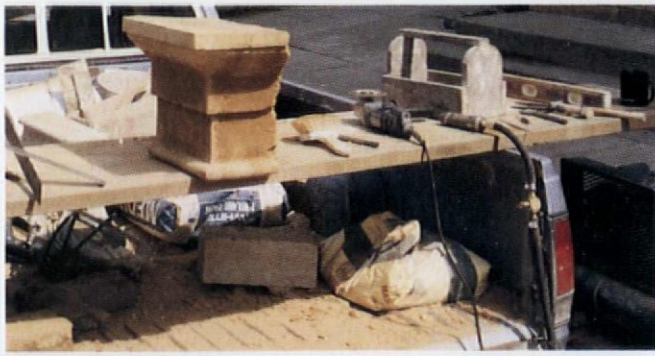
A nearly complete capital. Note the darker, inner stone that will change color and become uniform with the rest of the capital as the unit cures.
