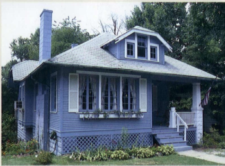
Top: Double-clipped gables identify this Pasadena home as a Pacific Ready-Cut. Bottom: This Sears "Hamilton" (1925-29) in Cheverly, Maryland, is a small hipped-roof cottage with jerkin-head dormers.
