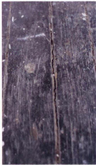
The cracks in this tongue-and-groove floor are actually dry-weather fissures in compacted dirt, which have opened to catch debris.
