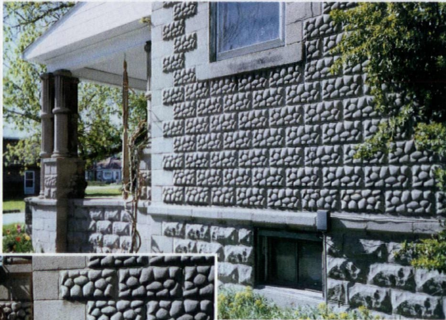
Mr. Whitman's house, pictured above, features an array of concrete-block effects, from smooth quoins to imitation stone; even the columns are concrete. The detail photo at left highlights the rock-face and cobblestone-face blocks.
