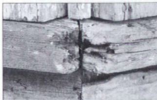
This rotted - and irreplaceable - woodwork...
