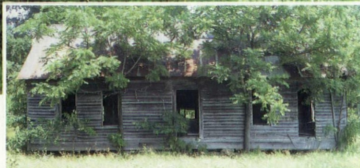
Board-frame construction remained a viable, and often preferred, building technique in White County through the 1930s. Pictured above is the Ike Wood House (circa 1890).
