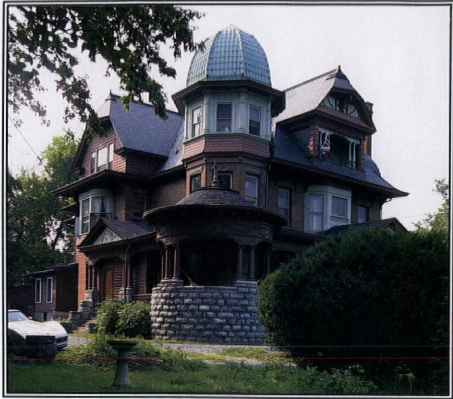
This house has the Barber touch — polygonal corner tower, jerkin-bead dormers, a mix of materials and Colonial Revival details like the swag decorations at the entrance and on the tower porch.
