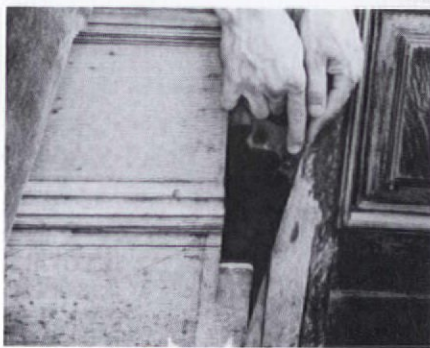
A small crosscut saw is tailor-made for trimming woodwork in tight or bidden places.
