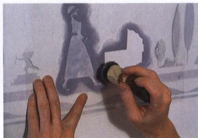
In a matter of seconds, the paint is applied using dry-brushing technique.
