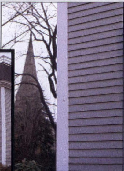
Buttolph Williams House, Wethersfield, Conn. (1692). Skived clapboard, 3 3/4-inch exposure.
