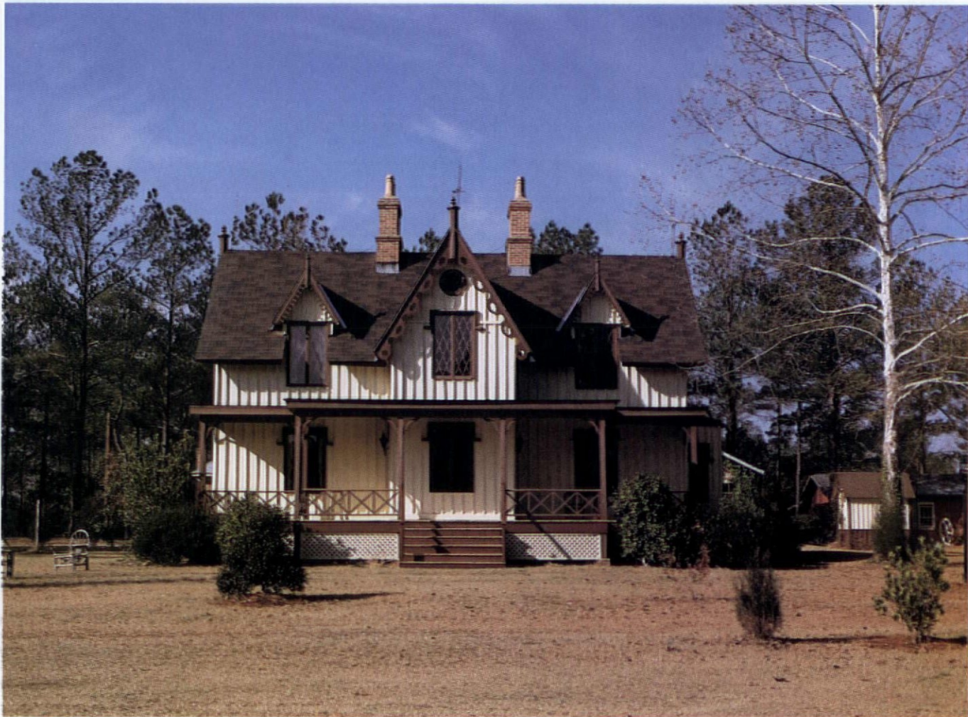
The cross gable was part of the original Downing plan. The full-width veranda and the gabled dormers were adapted from another Downing cottage. They help make south Alabama summers more livable.
