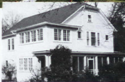
The Brentwood, from a later Aladdin catalog, shares elements such as the clipped gable and a sleeping porch with the Rices' house (inset).
