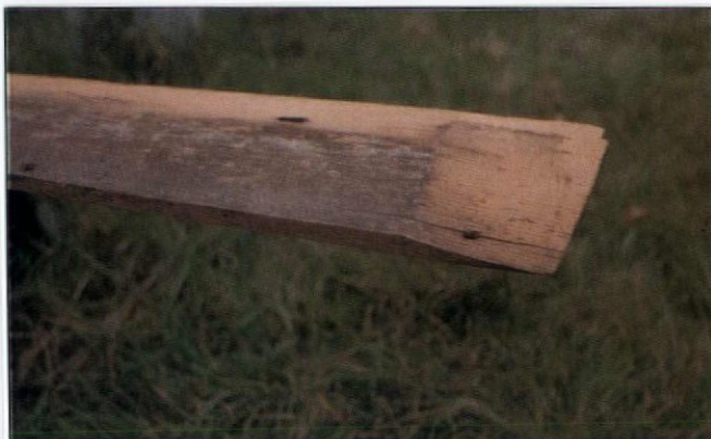
A band-rived and -skived clapboard (Reuben Ball House, Corinth, Maine, c. 1808). Note the two-course nail holes.
