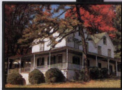
Buttolph Williams House, Wethersfield, Conn. (1692). Skived clapboard, 3 3/4-inch exposure.
