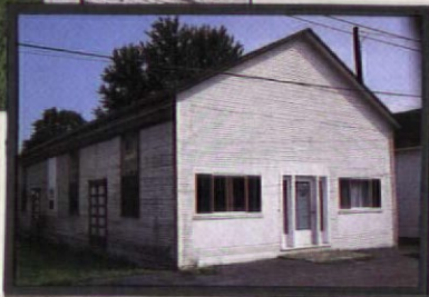
The ubiquitous "cove" pattern, also called "novelty" in its own right. Cove siding was popular by 1880, and may have been patented fifteen years earlier.
