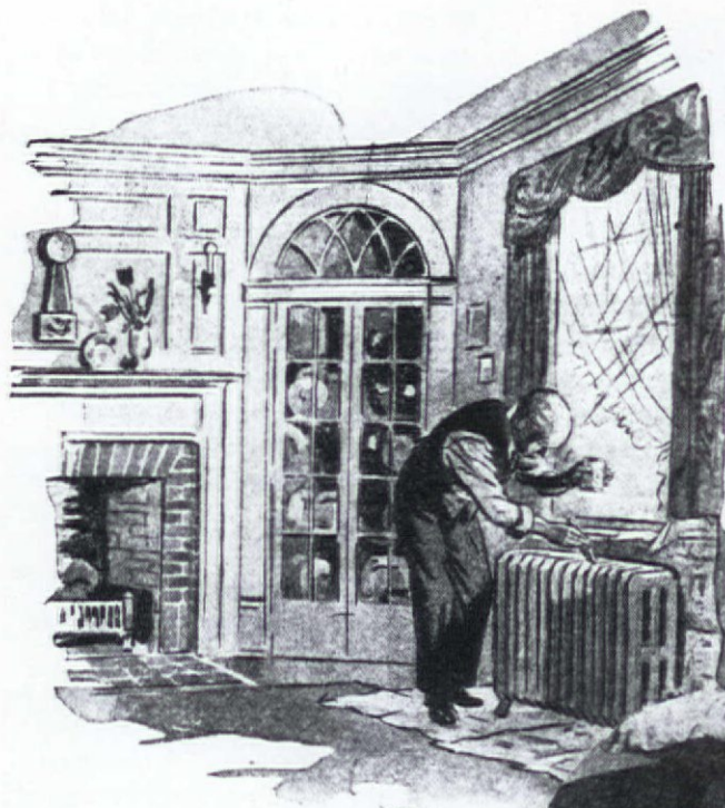
A base coat is applied to a radiator in a 1930 illustration from The Home Workshop Manual . Sponge stippling is shown in inset.
