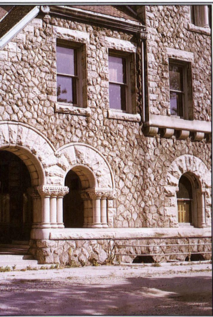
...Ives Cobb, architect. The entrance porch, with clustered ...Romanesque porches and porte-cocheres. ...stone walls is also typical of the style.
