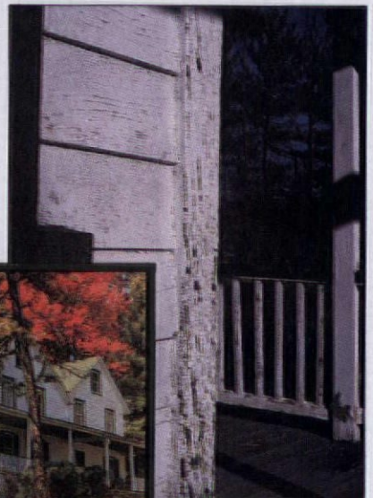
The Honold Homestead, Greeley, Penn. (c. 1880). Rectangular weatherboards, 4 1/2- to 5-inch exposure.
