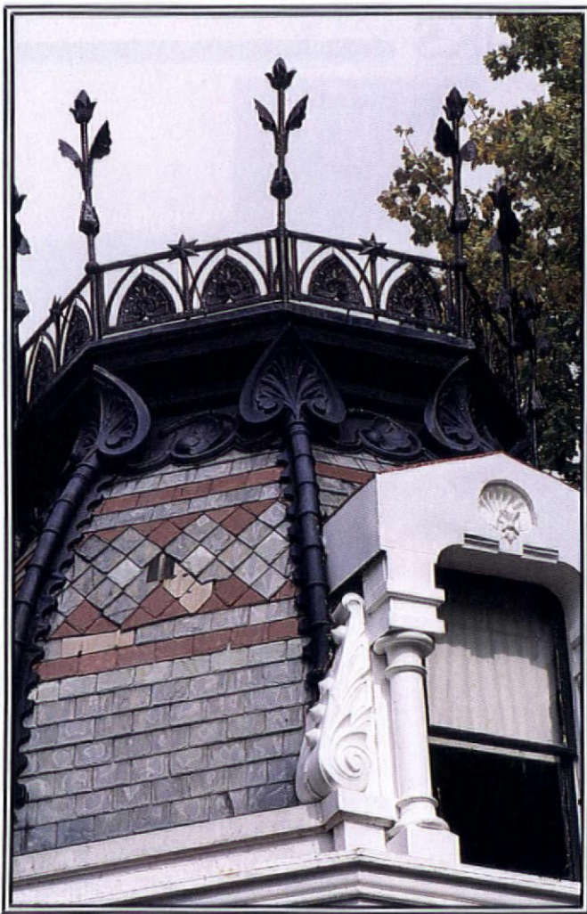
The height of fashion in a Second Empire house: a mansard roof in polychrome slate with cast-iron roof cresting.
