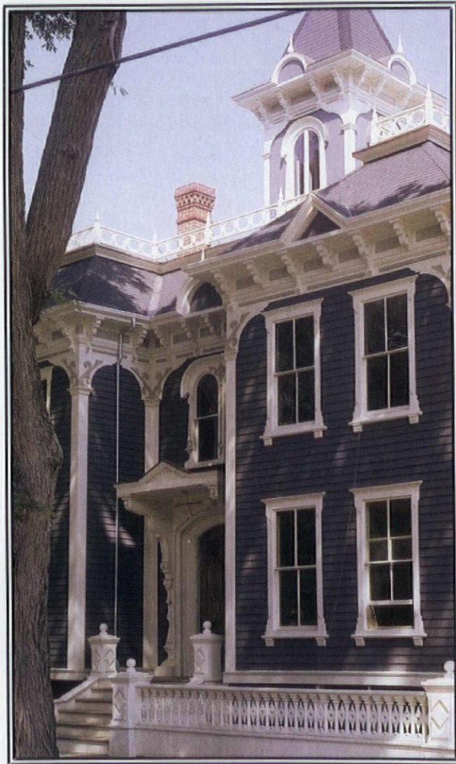
This house in Nantucket combines Italianate eave brackets, round arch windows, and a bell tower with a half-height mansard roof.
