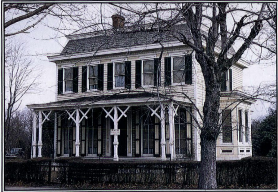
Most mansarded houses in America were made of wood, not stone or brick as were their French prototypes.
