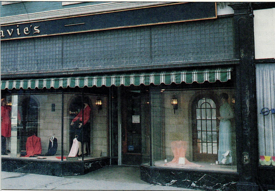
20th-century storefront: wide windows and transoms made of prism glass.
