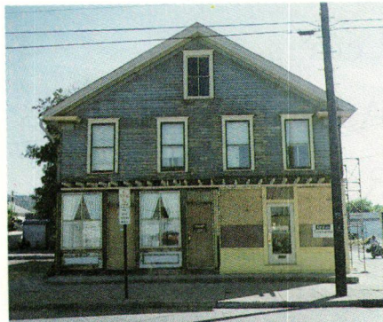
Many commercial buildings have been subjected to quick fixes rather than maintenance and repair. Sometimes just peeling off the coverups restores architectural integrity. (project: V. Romanoff & Associates, Ithaca, N.Y.)
