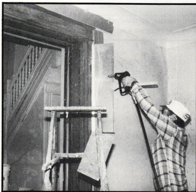
Besides full masking, the operator uses a shield to control overspray during pressure rinse. (Photos courtesy of Bix, except as noted.)
