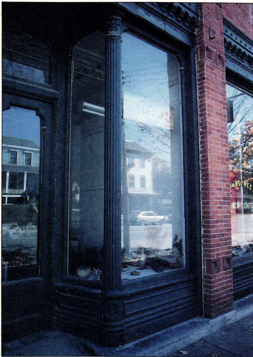
A smashing combination: late-19th-century cast iron and polished plate glass.
