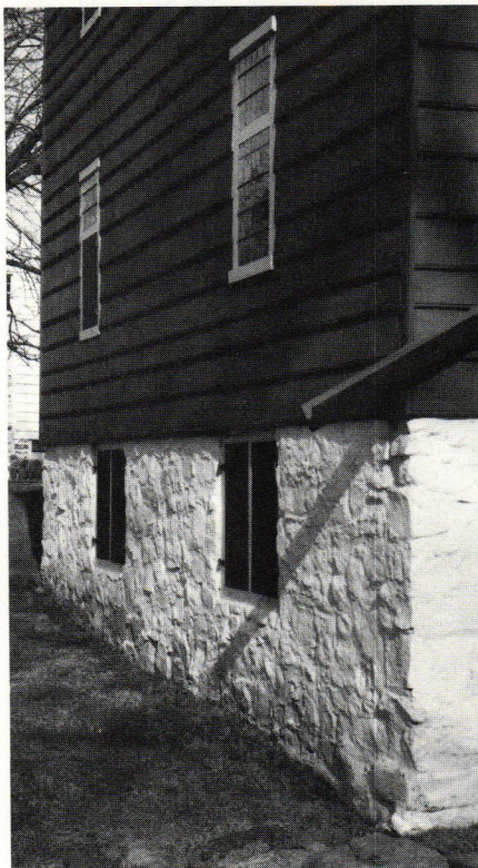
Hand-mixed paint and whitewash at Richmondtown, Staten Island, N.Y.
