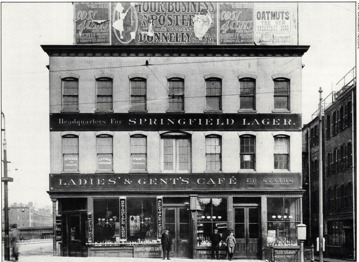
Shop-window evolution in a Boston storefront: a plate-glass retrofit, left, and an earlier two-over-two design, right. (c. 1900)
