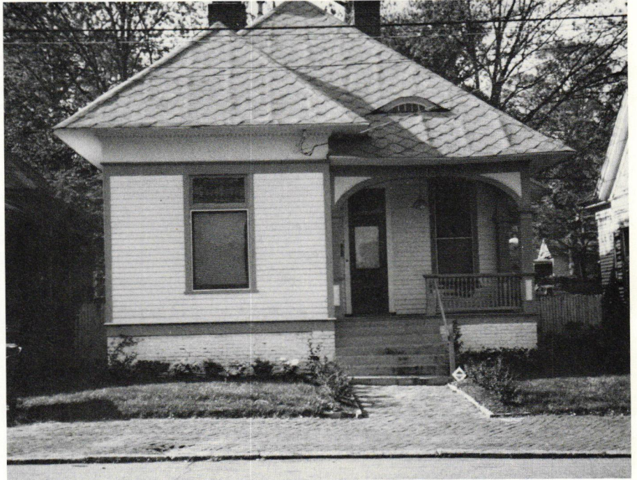
A simple Victorian Cottage in Atlanta.
