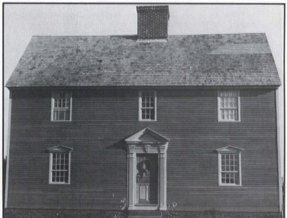
The Bronson Homestead (1860-1740) — a restoration, but with all new exterior millwork.
