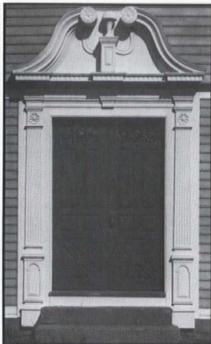
Correct 18th-century Connecticut River Valley millwork.
