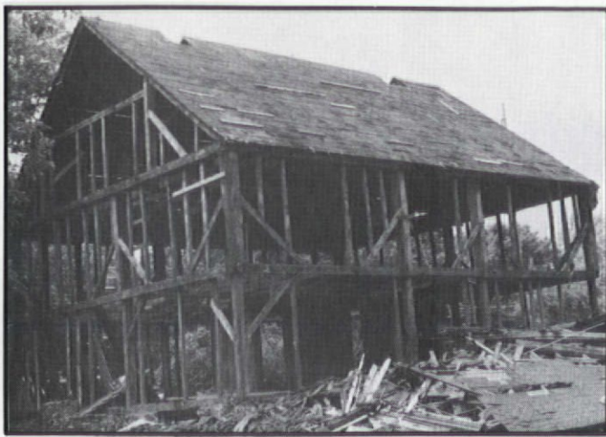
The Benjamin Moore house during disassembly.
