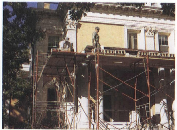
Terra-cotta restoration underway at the Grant-Humphreys Mansion.
