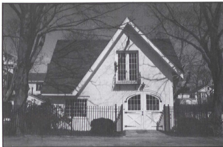
This is the side-street view of the carriage house above. The first storey, authentic on the interior, houses antique autos; above is a guest suite.
