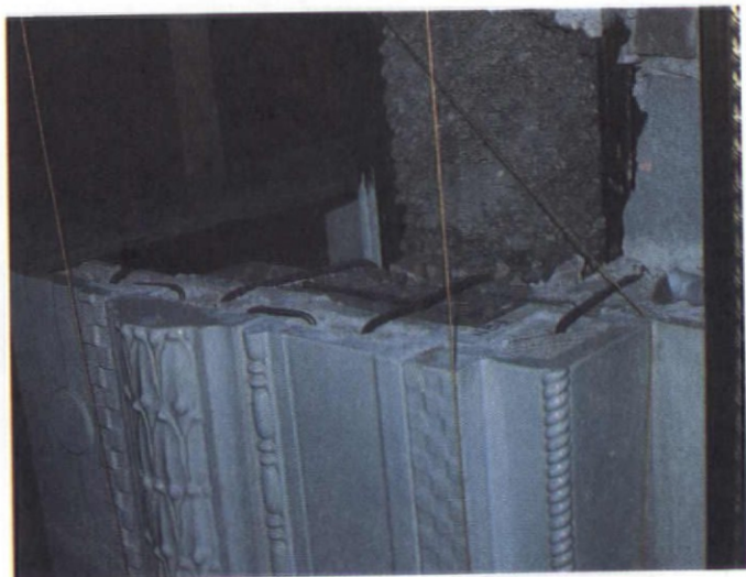
Installation of new terra cotta. Note complex anchoring system.
