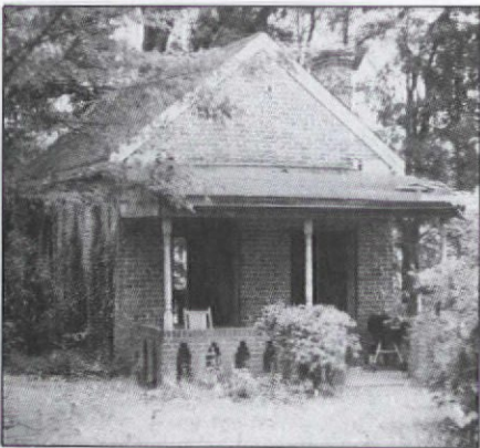
This old brick house (above) in North Carolina was cleaned by water-blasting; but will it do the trick for this outbuilding (below)?
