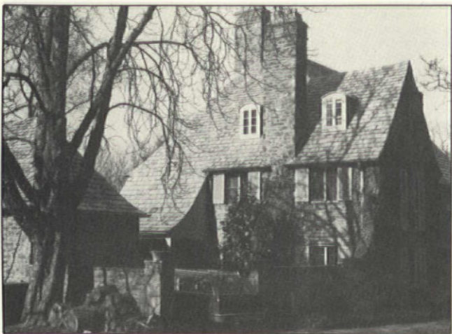
The garage is incorporated into this French Norman house's walled "compound," an imitation of medieval gathered outbuildings.
