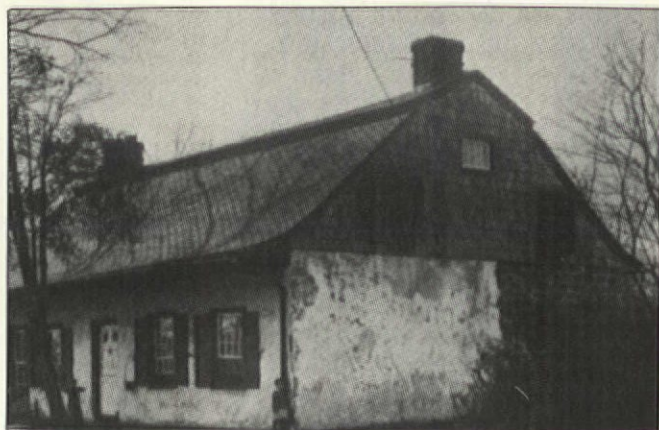
Dutch house with overhanging eaves, Bergen County, N.J.
