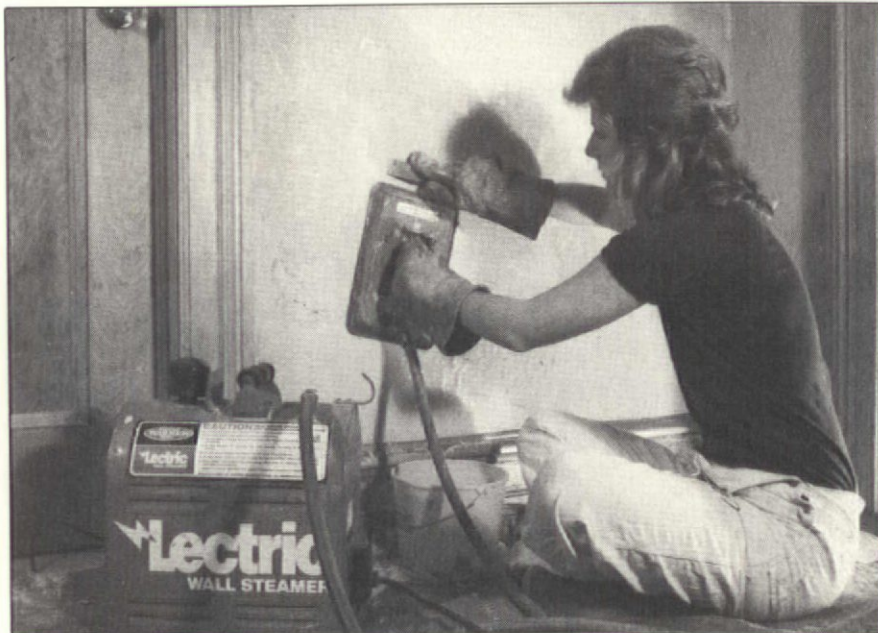
Spending the day with a wall steamer and putty knife is no joy, but these simple tools will remove most texture finishes effectively.
