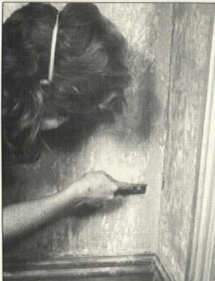
Use a "combat chisel" on the remaining finish.
