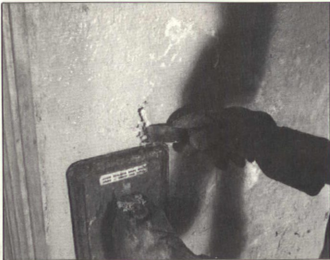
The finish falls off in wet chunks -- no dust is created.
