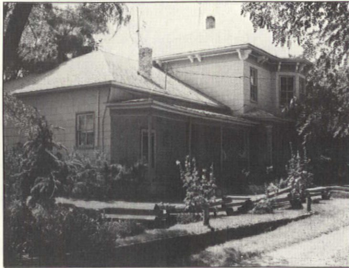
When resources allow, David and Millie Moore (seen standing, like their ancestors, on the front porch) are going to remove the asbestos siding.
