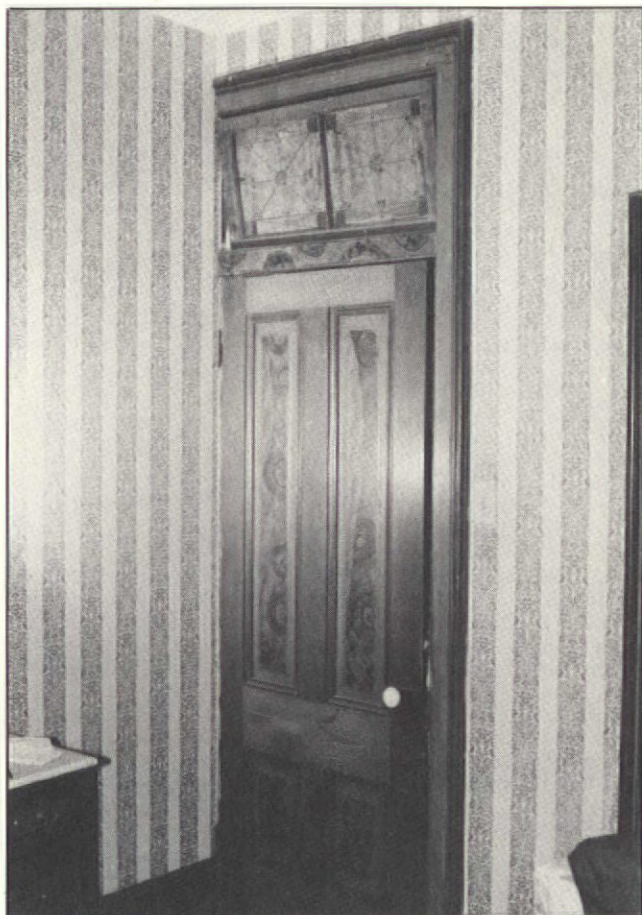
Every door in the house has a transom painted with a geometric design. This door, in the bay bedroom, also has its original painted grain.
