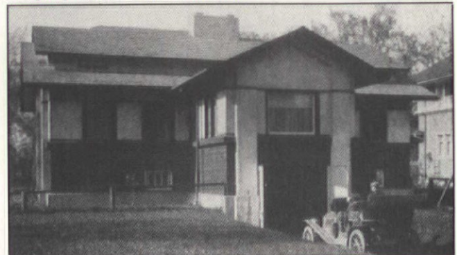
This circa 1921 house contains a very early example of an integral garage; the plan book in which it appears calls the building "an interesting suburban home with a garage in the basement."
