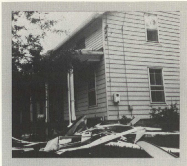
Shorn siding lay in heaps around the house.
