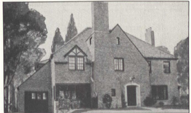
The irregular rooflines of Tudor Revival homes lent themselves to integral garages, as on this 1926 house.
