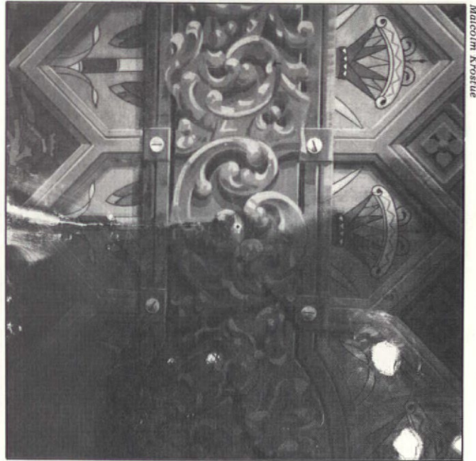
Dirty glaze is removed from a decorative painting in Michigan's Honolulu House (Hasbrouck Hunderman, Restoration Arch.).
