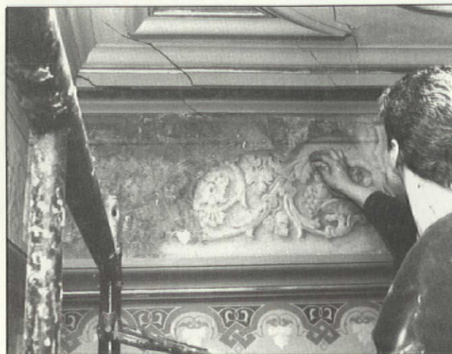
. . . as Darla washes down the area with a hot-water-and-vinegar solution, the frieze returns to elegant life.
