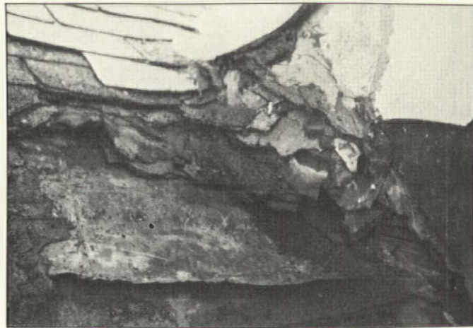
So many layers of roofing — but none of them could save the bathroom ceiling.
