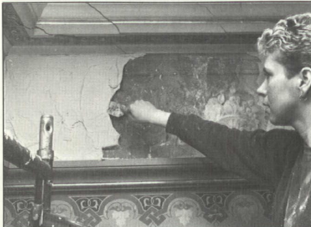
Darla Olson removes the poultice — the surface seems as dirty as before, but . . .
