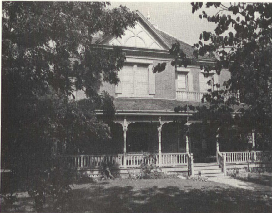
Here's a close-up of the front (east) facade.
