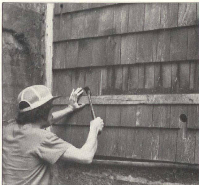
Above: Shingles in the final course may not fit full length. Trim the top by the distance the shingle sticks out at the bottom. Below: One way to keep the course line straight.
