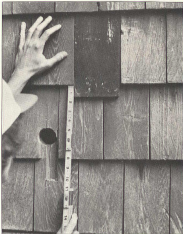
Above: Shingles in the final course may not fit full length. Trim the top by the distance the shingle sticks out at the bottom. Below: One way to keep the course line straight.
