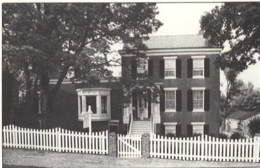
Gibson Hall, built in 1832, was acquired by a group of Washington, D.C., investors in 1983. In the heart of Virginia's hunt country, the heavily renovated inn provides such up-scale amenities as queen-size beds, skylights, and private baths with sunken tubs and jacuzzis -- a far cry from the down-the-hall facilities of most home-style bed-and-breakfasts. A small mortgage, relatively low interest rates, and many investors put the inn in a better position than most to withstand high renovation costs and inevitable seasonal lags in rental income.
