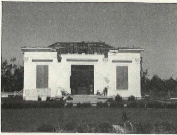
The house after the June 3, 1980, tornado — decapitated and windows boarded.
