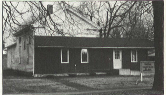
The remuddled Greek Revival in Rockford, Illinois.
