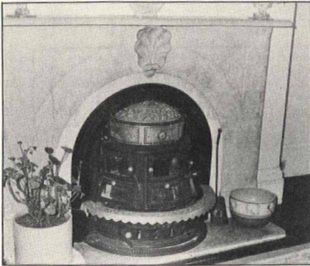
Left: The 'Grand Heater' was the top of the line at Baltimore's Sexton Stove Company. Note the nickel-plated filigree trim, the plated knobs, and the plated foot-rest of this restored Grand. An art tile medallion decorates the stove's crown. The filigree dome atop the
