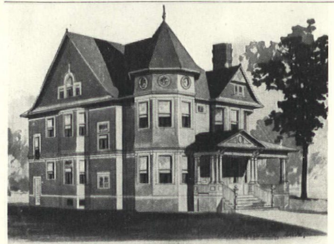
This 1903 Neo-Colonial has the asymmetry of the typical late Victorian Queen Anne, but also includes a Palladian window and a pedimented porch with Doric columns — symbols of the newly fashionable "old colonial" style.
