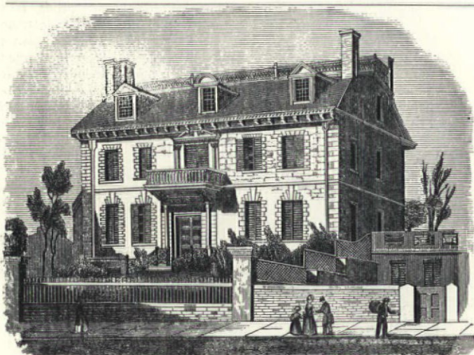
A full set of measured drawings of the Hancock house in Boston (built 1740) was made before the house was demolished in 1863. In the 1890s, these drawings became a source of inspiration for the champions of the Colonial Revival style.
