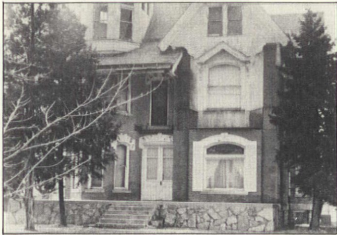
Left: This is how the world saw the Boesel house prior to the Kucks' rescue operation. (The house looks really naked with-
